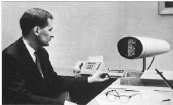
1965 As a result of earlier trials, significant equipment and operational changes were made in the Picturephone system. The modified equipment was used in a product trial begun in July 1965, in cooperation with Union Carbide Corporation. In December of the same year an experimental trial began at AT&T headquarters in New York City. In June, 1967, the trial was expanded to include three Bell Labs locations. This trial integrated Picturephone service with normal telephone service. This "corporate network" offered an opportunity to explore additional uses for the system, such as the feasibility of using the Picturephone set as an interface between man and computer (shown here). The computer is interrogated from a Touch-Tone® dial, and results are displayed on the screen.
