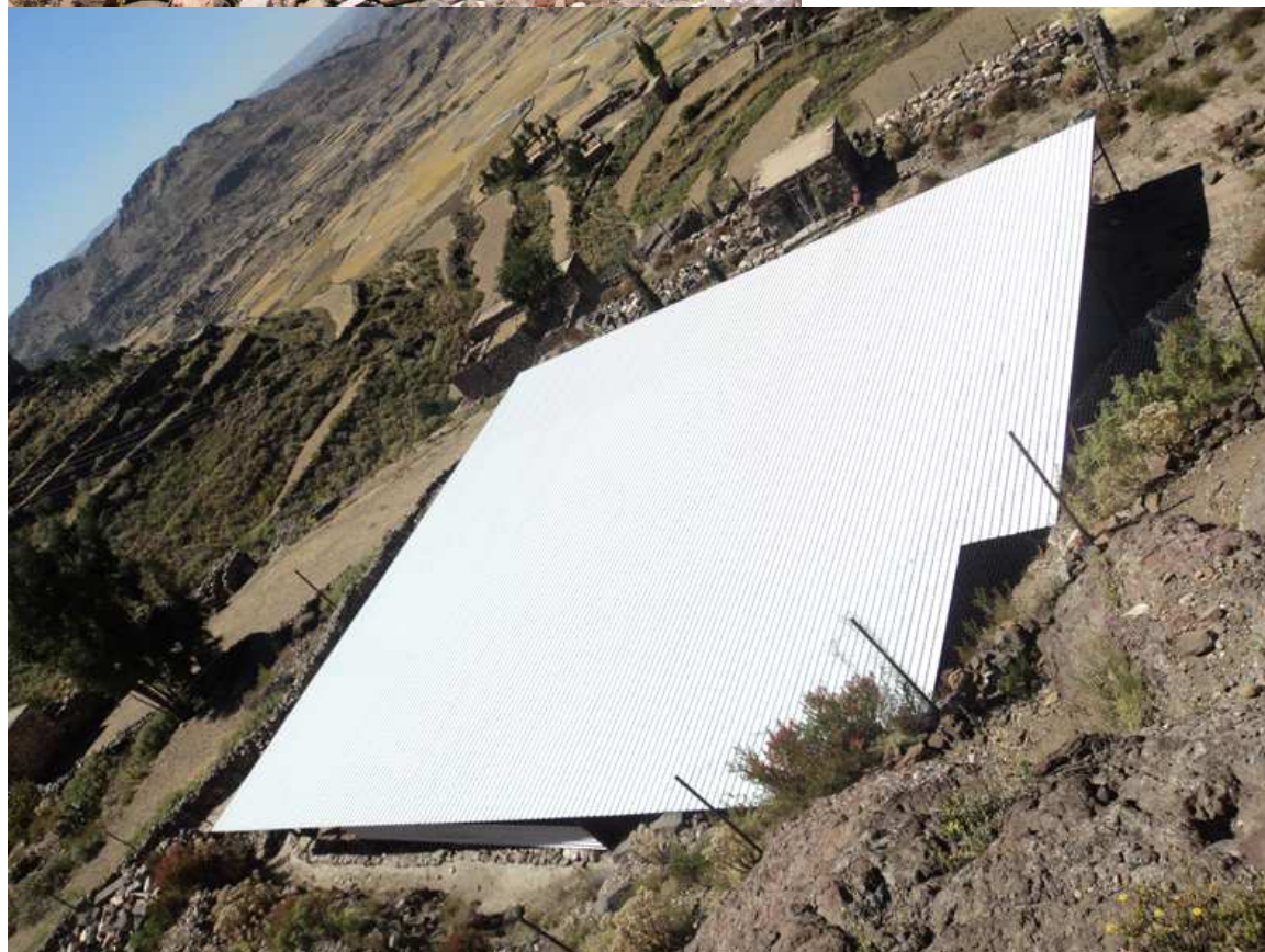
Fig. 2. New roof over the entire Himyarite period Stone Building.
