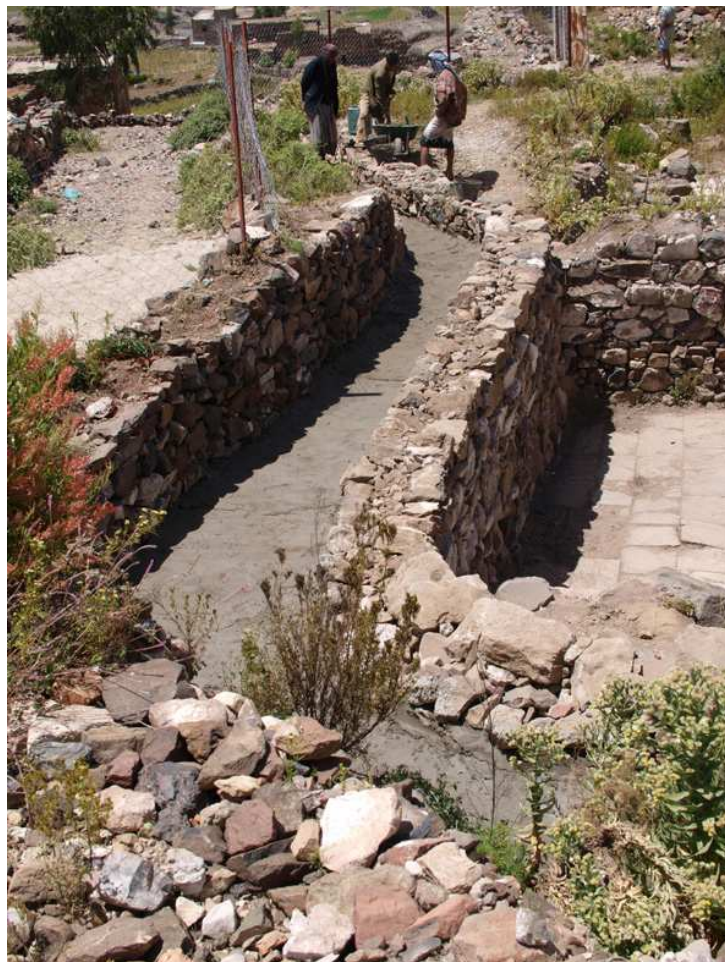
Fig. 1 The new water channel in the Stone Building.
