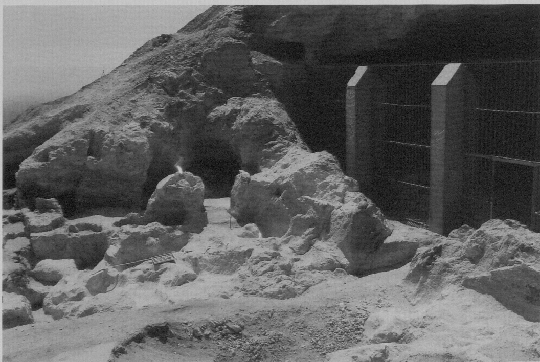
Tomb III, forecourt: remains of southern part of the front wall and entrance to southern side chamber
