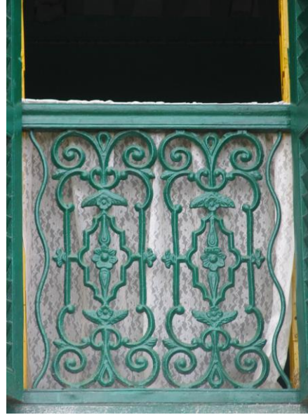
Fig. 189 Patan, Naṭol: Precast iron ceiling of an Amatya house (after 1934). The pattern was the model for carved wooden ceilings.
