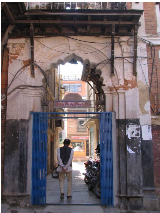
Fig. 82 Wanabāhā, Patan: The gateway presents a Mughal multifoil arch enclosed by a neoclassical blind arch with trapezoid keystone and framed by Corinthian pilasters.
