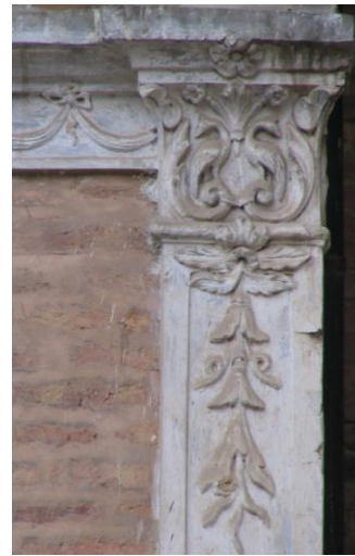
Fig. 331 The pilasters in the first floor are adorned by two birds that frame a flower vase, like fish frame the auspicious vase in Buddhist tradition. The façade is built with unglazed bricks ( māpā ) and lime putty.
