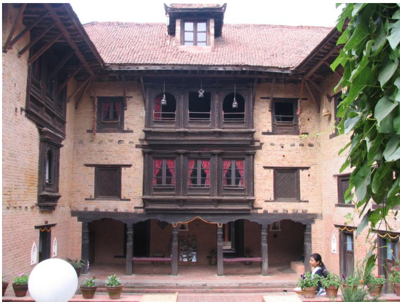
Fig. 4 Patan, locality of Svatha: Symmetrical courtyard-façade of a renovated Shrestha house from early Shah period. It is built of brick and wood although there are no signs of a European form language yet.
