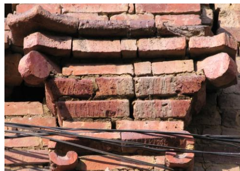
Fig. 590 Brick capital based on the Ionic capital on the first floor. The bricks were trimmed and arranged in eight layers.
