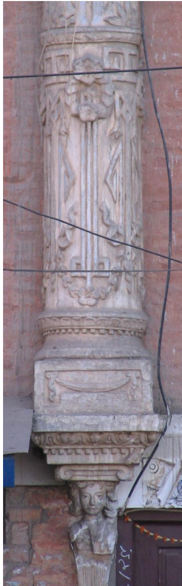
Fig. 351, 352 The colossal half-columns are borne by consoles in the form of caryatides. The shafts are adorned by Art-Nouveau design.
