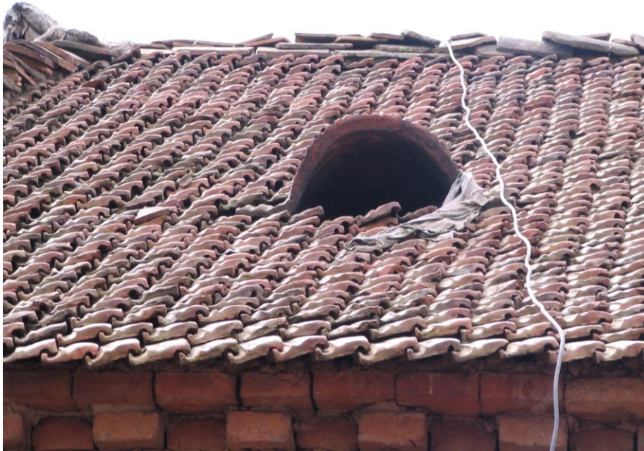
Fig. 36 Roof openings for light and ventilation ( bhaugāḥ ) are covered by specially-moulded, round tiles. The firing with rice straw was only possible on the roof level, because the smoke could easily escape through these so-called “cat-holes”.
