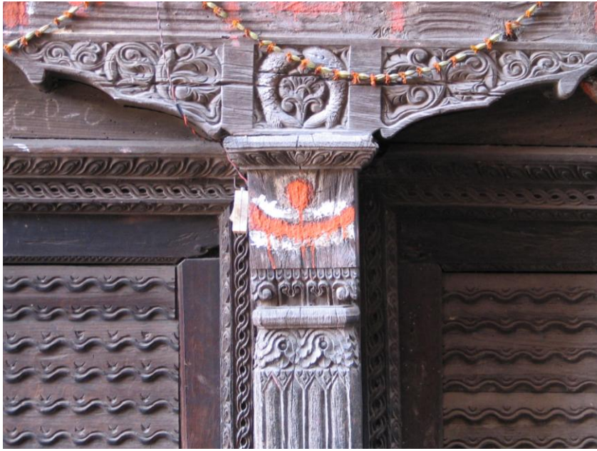
Fig. 19 Bhaktapur: Late 19 th century capital made of one piece: The capital is characterised by the diminution of its cantilever and is typical for Newar load-bearing constructions. A pair of fish ( suvarnamatsya ), one of the eight auspicious signs ( aṣṭamaṅgala ), adorns the cube, while the cantilevers are embellished by lotus scrolls. A plate is set between the shaft and the capital. The shaft is adorned by the Newar interpretation of the acanthus motif ( desisvā ) below corner volutes ( sāythū ) and a torc ( nāḥgvaḥ ).
