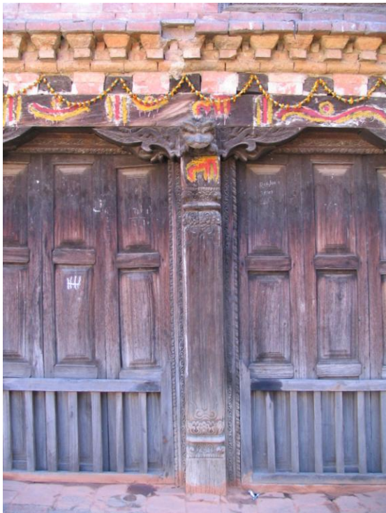
Fig. 20 Bhaktapur: The part of the ground floor that turns to the street or courtyard opens up with a row of wooden pillars. The pillars and capitals may be decorated by a great variety of patterns. The cube at an early 20 th century house has the shape of a mythical animal ( kūsuru ) and the cantilevers are carved in the shape of dragons ( malah ). Auspicious symbols are painted on the lintel.
