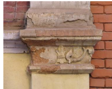
Fig. 230 Patan, House in Svatha: The Tuscan capitals in the ground floor are adorned by lotus arabesques. The design is stuck on the plaster made of brick dust (chun-surkhi) and quick lime.
