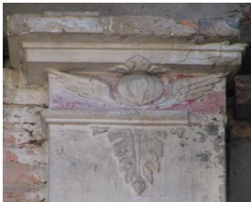
Fig. 228 Patan, house at Nalachibāhā: The capitals in the 2 nd floor resemble the Tuscan order. They are adorned by an ornament based on the Egyptian sun symbol while the shaft is embellished by acanthus.
