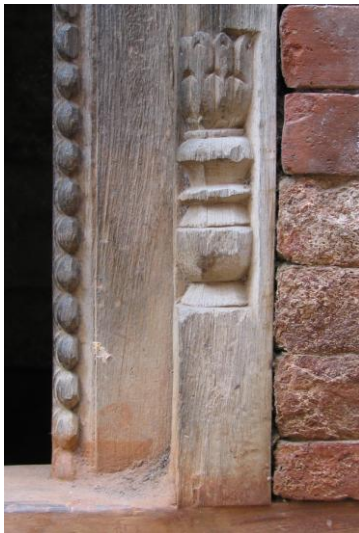
Fig. 579 Detail of the door: Vase-like element with lotus leaf design at the bottom of the colonnette. The inner door frame is embellished by walnut pattern ( khvāṣī ).
