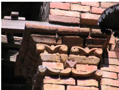
Fig. 275, 276, 277, 278 Bhaktapur: Variety of brick capitals. Protruding worked brick stones in the form of two symmetrically arranged bricks trimmed in cambered form with small volutes on each end. The abacus exists of layers of brick. Beaked corner-eaves tiles ( gvāgaḥcā ) are characteristic Newar features. Whereas motifs like a heart are rarities, traditional patterns like the kaṣimvahaṇā , a brick frieze with lotus leaf pattern ( palehaṇā ) are often used to adorn the capitals.
