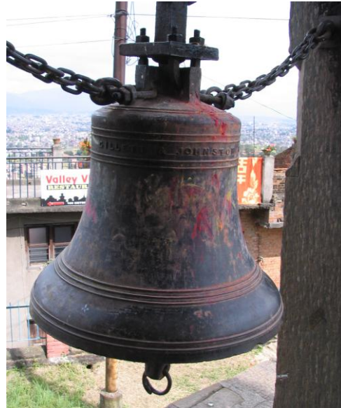
Fig. 215 Kirtipur, Uma Maheshvara temple: Tall, heavy, iron bell from “Gillet & Johnston Founders Croydon 1895”. It was originally a quarter- striking bell from the Ghanta Ghar clock tower, Kathmandu.
