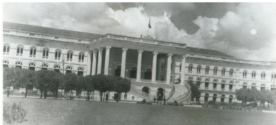
Fig. 99: Photo from the 1920s. The towers were removed and the two pairs of buildings were covered by a continuous ridged roof. A semi-circular gallery based on the design of the Government House in Calcutta was added to Nārayanhiti, but only at one corner of the building. A split, double staircase, also found at Kedleston Hall, England, was another addition to the building. Sources: Kathmandu Valley Preservation Trust.
