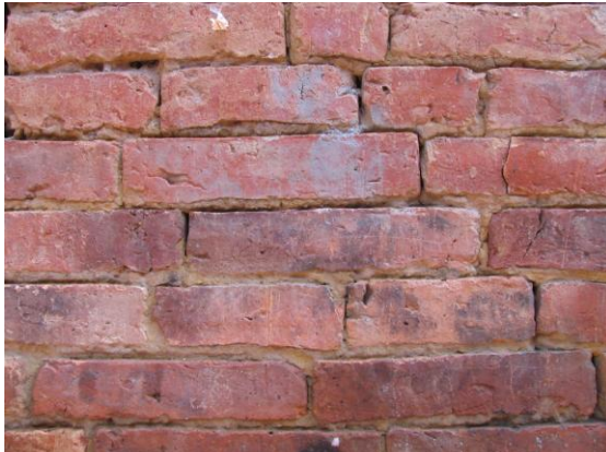
Fig. 22 The façade of a Newar house is either built of burnt brick, māapā , (above), or dātiapā (right) with a red scumble on its front side.
