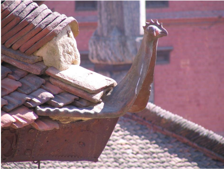
Fig. 35 Beside the rectangular roof tiles ( āypā ) the roof-like kvapuapā cover the hip-ridge. The corner-eaves tiles may be embellished on their cusp by the head of a rooster.
