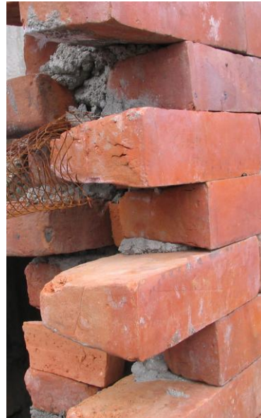
Fig. 23 The dātiapā with a red scumble on its front side is a conical veneer brick that produces flush joists.
