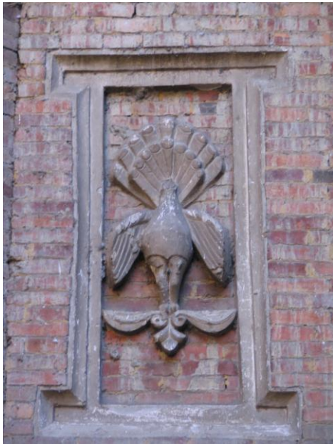
Fig. 419 Bhaktapur, Jēlā: The blind window takes up the format of a Newar early 20 th century window. The window frame is plastered and the peacock moulded in stucco.
