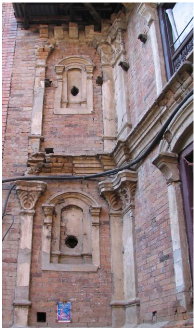
Fig. 72, 73, 74 Bhaktapur, Kvāchē: Wooden miniature blind window ( dyahjhyāḥ ). Instead of being closed by an apron plank the bust of a deity looks out. Bhaktapur, Chochē: The Mughal-style blind niche with an ogee arch and with a stucco frame in the first floor is the focus of the façade. Bhaktapur, Tāpālāchē: Neoclassical blind windows in the first and second floor are rendered while god-holes ( dyahpvāḥ ) are left for the passage of spirits.
