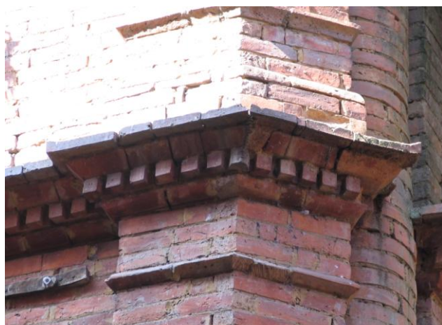
Fig. 279, 280, 281 Bhaktapur: Variations of protruding worked brick stones with small volutes on each end, arranged symmetrically. A brick is worked in the form of a drop dangling from the centre. Protruding and worked bricks mark the astragal. The abacus exists of four layers of bricks, partly arranged to form a dentilation and partly as half as thin as the model brick used for the façade. Beaked corner eaves tiles ( gvāgaḥcā ) are characteristic of most brick capitals.
