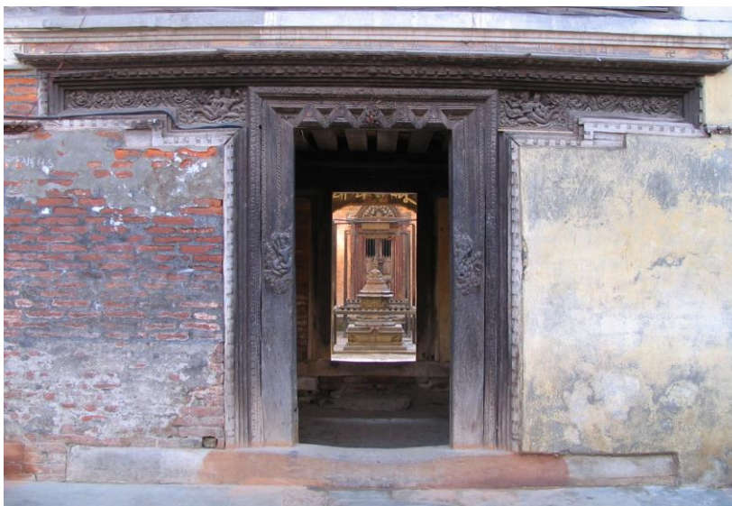
Fig. 24 Patan, Gujībāhā: The threshold and lintels are special characteristics of the Newar way of construction: They project beyond the jambs and remain visible in the wall. The frame with long wooden sills and lintels bears artistic carvings and the lintel's dentil (or teeth) pattern that presents an uneven number of trapezoids is considered to be an auspicious symbol.
