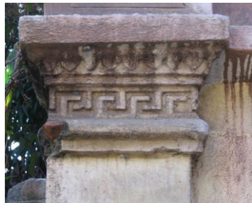
Fig. 229 Patan, house near Valakhu: The Tuscan capitals are embellished by meander design.
