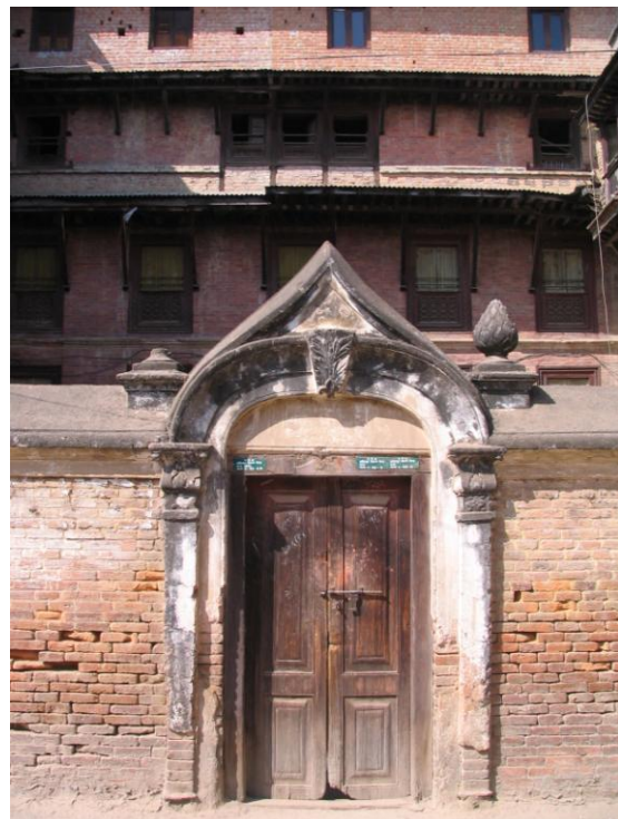
Fig. 83 Patan, Caki: An ogee arch, characteristic for Islamic architecture, is found above the portals of an entrance gate. Neoclassical pine cones beside.
