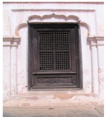
Fig. 70 Detail of Lal Baithak: A Moorish multifoil arch spans a Europeanised Newar lattice window with crossbars. The upper storey was dismantled after the earthquake in 1934.
