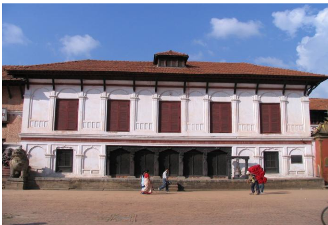
Fig. 69 Bhaktapur, Darbār, Lal Baithak (c. 1870): The façade combines the Mughal design of the blind windows with a re-used Malla-period arcade in the ground floor.
