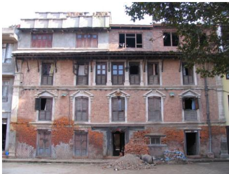
Fig. 370 Characteristic Newar alignment of the openings in the ground floor with a huge entrance of a passage in the centre. The generous façade offers enough space for a modern version of a window with five openings rarely found on 19 th century buildings.
