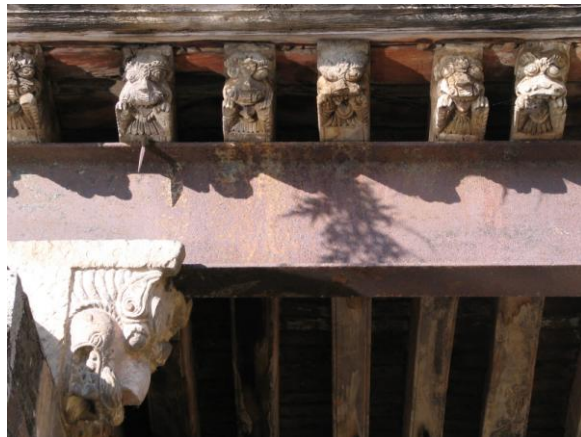
Fig. 217 The bridge (1913) is constructed of massive piers made of bricks and is borne by rolled girders from world famous Dorman Long, Middlesborough, England. Decorative stone consoles with lion faces support the heavy beams. Wooden joists are laid across their ends being carved ( dhalīmvaḥ ) in the shape of typical Newar mythical animal's faces ( kūsuru ). They are covered by bricks.
