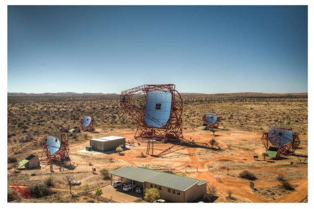
**Figure 3.2:** Aerial view of the full HESS-II array. In front of every telescope is a camera shelter, where the camera is parked during time of non operation. At the bottom of the image is building with the control rooms and the mechanic's and electrical workshops. Image credit: Christian Föhr.
