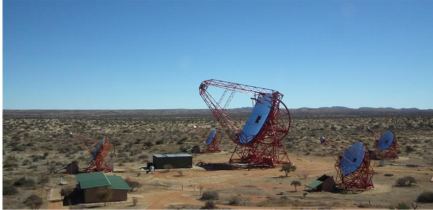
Figure 2.7: The H.E.S.S. experiment in its second phase, showing all five telescopes, taken from the official H.E.S.S. website [29]. The fifth telescope situated in the centre of the array has  $\sim 6\times$  the mirror area of one of the smaller telescopes.
