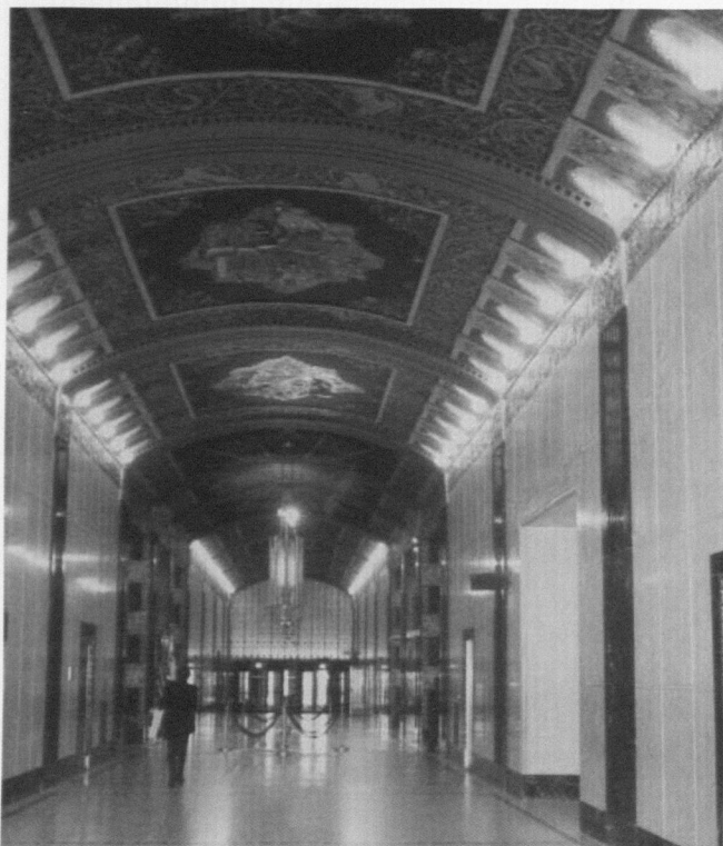
8. Nowy Jork, Barclay-Vesey Building. R. Walker, McKenzie, Voorhees & Gmelin, 1923–1926. 140 West Street. Fot. I. Grzesiuk-Olszewska
