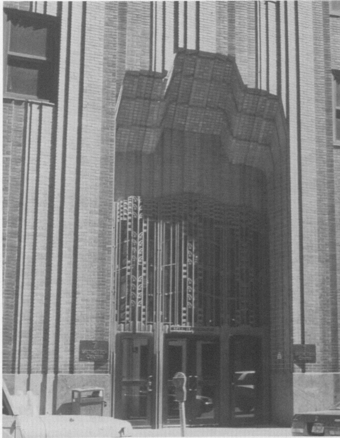
24. Nowy Jork, Brooklyn, Telephone Building, Voorheese, Gmelin & Walker, 1931. 95 Willoughby Street. Fot. A. K. Olszewski
