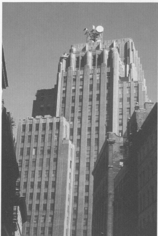
14. Nowy Jork, Long Lines Building, R. Walker, Voorhees & Gmelin, 1918, 1930–1932. 32 Sixth Avenue. Fot. A. K. Olszewski
