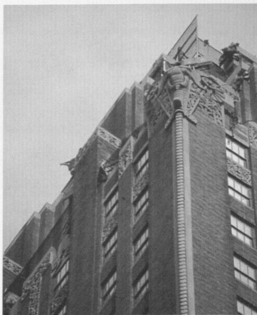
7. Nowy Jork, Barclay-Vesey Telephone Building, R. Walker, McKenzie, Voorhees & Gmelin, 1923–1926. 140 West Street. Fot. A. K. Olszewski
