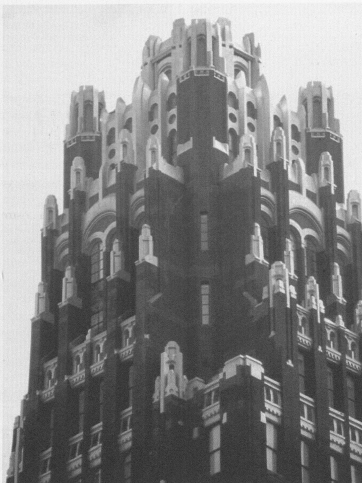
29. Nowy Jork, American Radiator Building, R. Hood & A. Foulhoux, 1924, 1937. 40 West 40 Street. Fot. A. K. Olszewski
