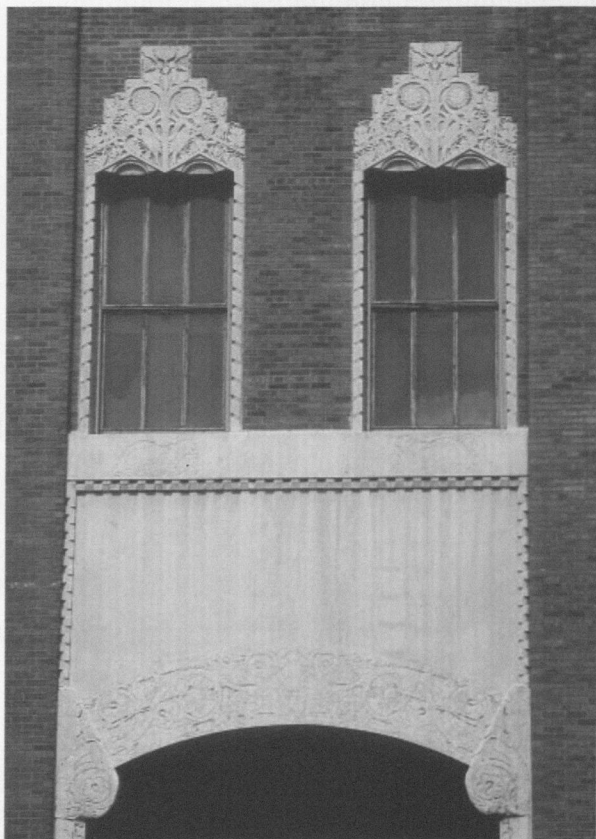
6. Nowy Jork, Barclay-Vesey Telephone Building, R. Walker, McKenzie, Voorhees & Gmelin, 1923–1926. 140 West Street. Fot. A. K. Olszewski
