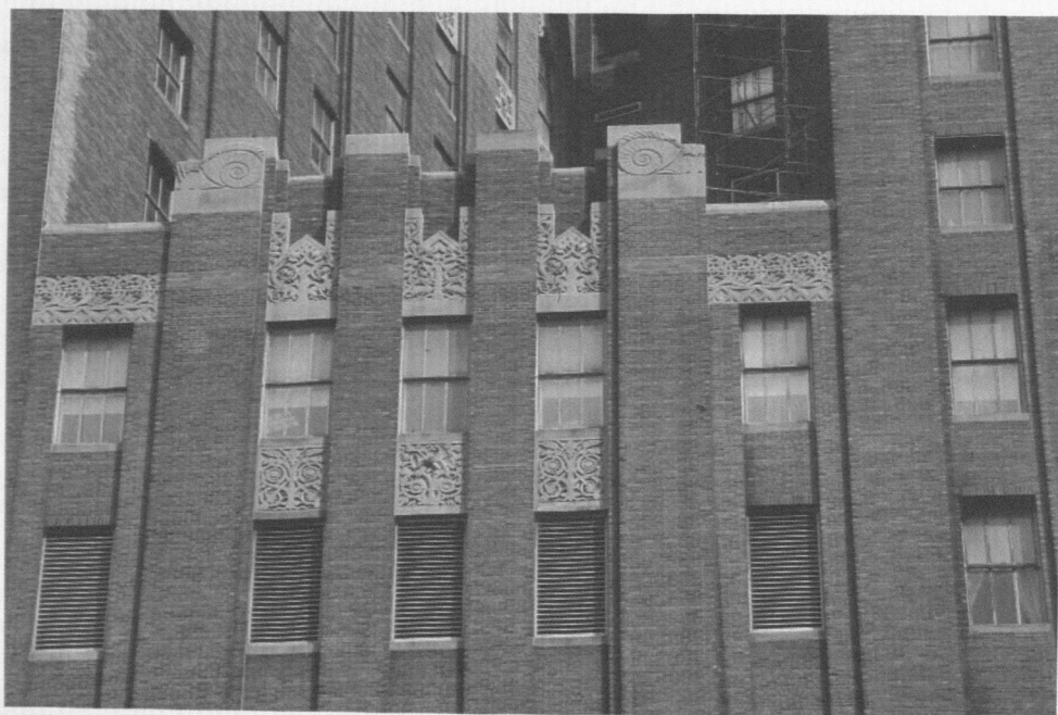
5. Nowy Jork, Barclay-Vesey Telephone Building, R. Walker, McKenzie, Voorhees & Gmelin, 1923–1926. 140 West Street. Fot. A. K. Olszewski
