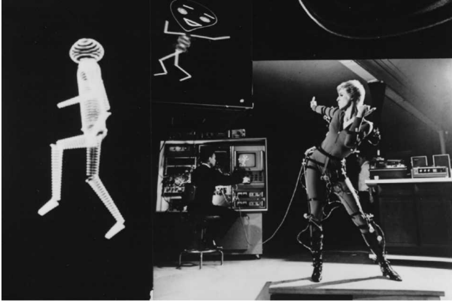
Harrison III, Lee: ANIMAC, 1962. A dancer controls the line patterns of a figure by activating sensors mounted on her body. Denver 1962 (photomontage).
