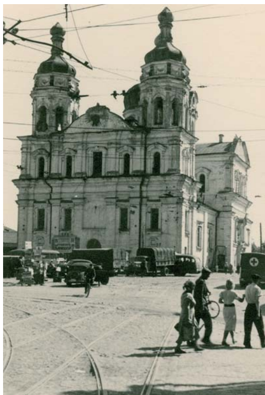
Fig. 16. Witebsk, 1712-1731 (destroyed 1944). Archival photo 1941, from the collection of Jakub Kotowicz.
