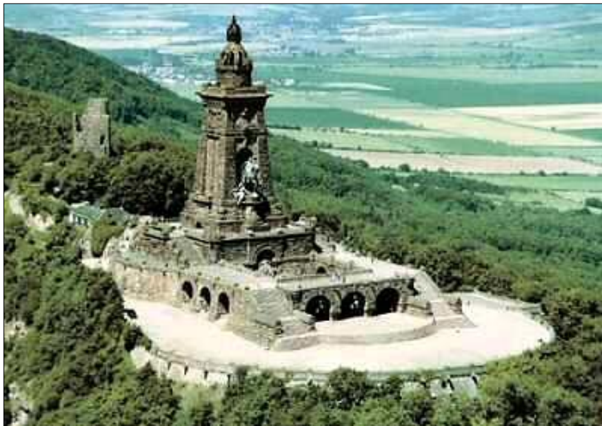
Fig. 48. Two views of the Kyffhäuser monument.
