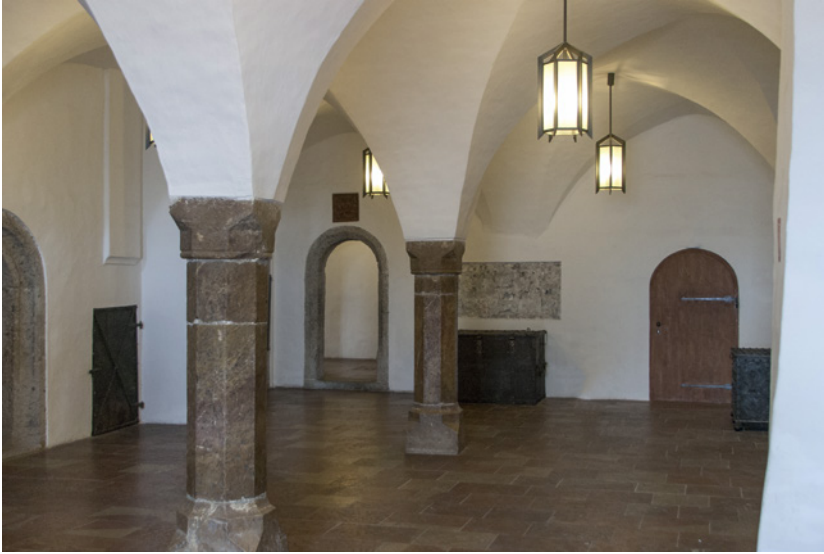
FIGURE 19.8 Hohensalzburg Palace at Salzburg, central staircase hall with a Romanesque Renaissance vault (ca. 1480–1485)
