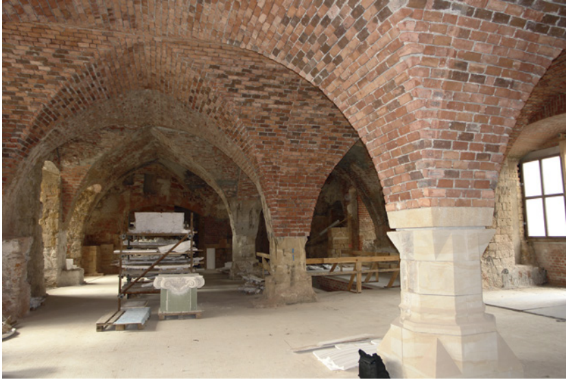
FIGURE 19.3 Arnold of Westfalen (attributed), Dresden, Schloss, ground floor hall of the east wing with its Romanesque Renaissance vault, so called “Gotische Halle” (ca. 1470–1475)
