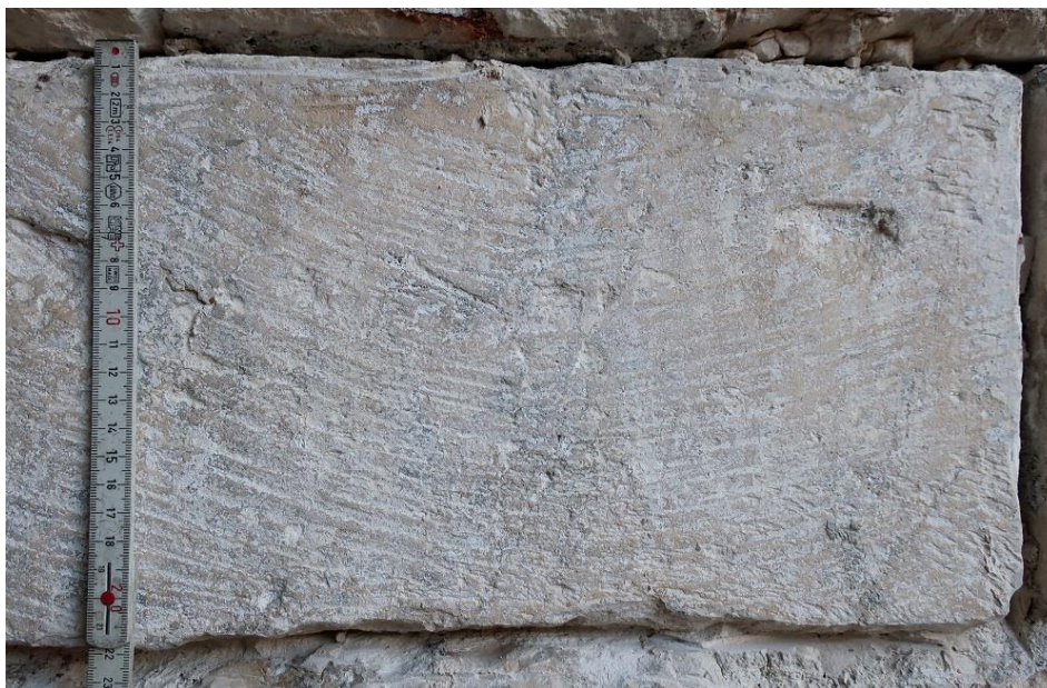
Fig. 6 - Cloister of S. Maria Latina (today Church of the Redeemer), example of surface treatment of stone blocks (photo: Dorothee Heinzelmänn, 2019).
