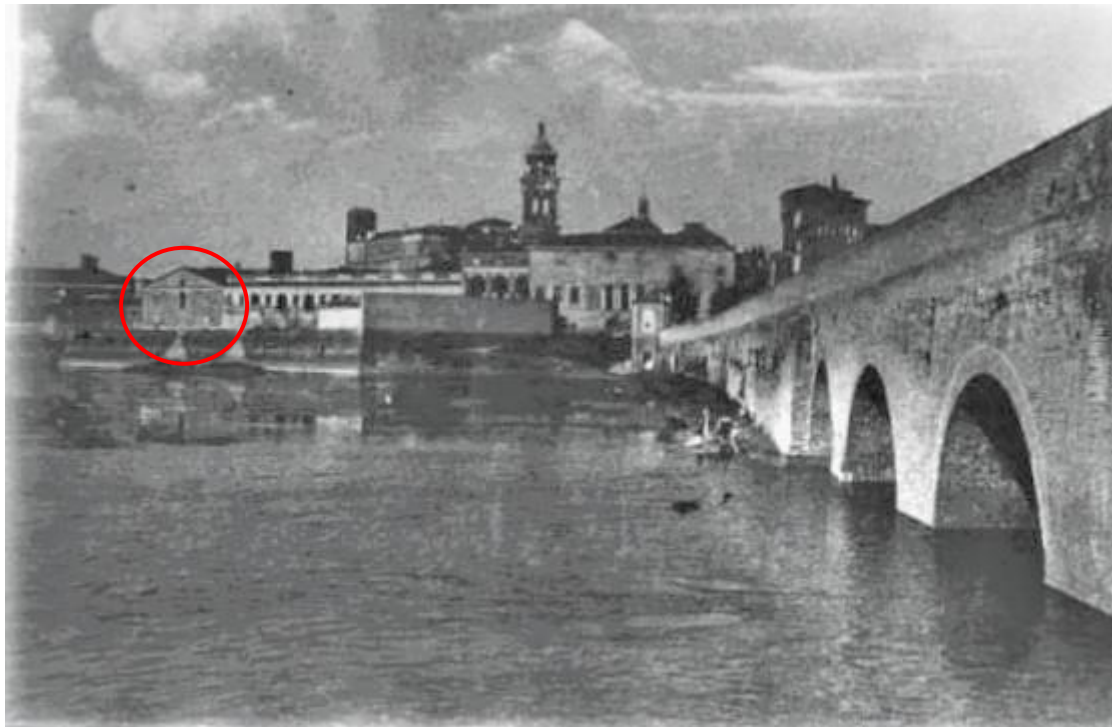
Fig. 13: The Ponte San Giorgio before the demolition of the bridge and the new construction at the end of the 19th century with a view of the Palazzo Ducale in red marks the Rustica with the old bridge on the right.
