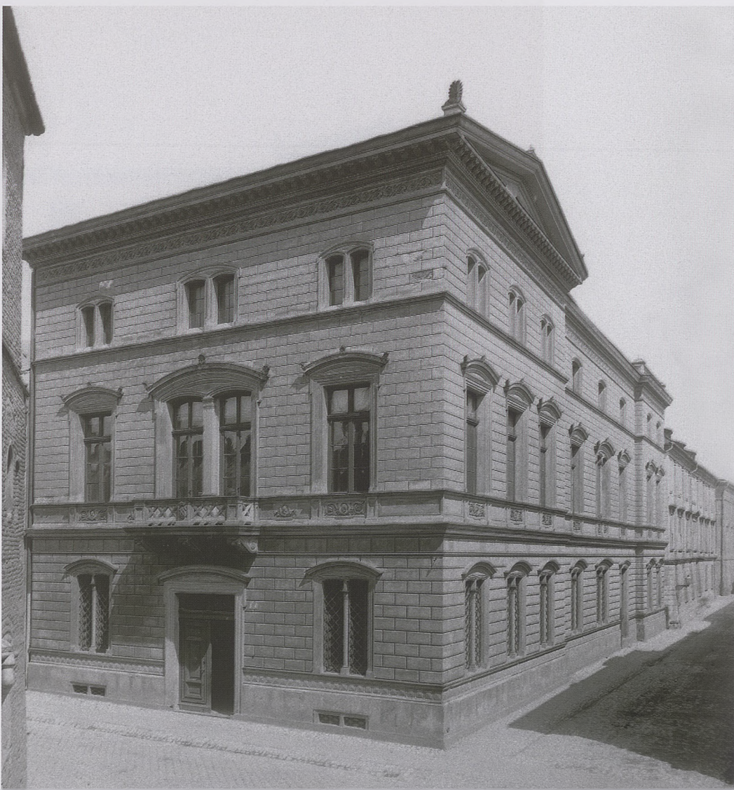
14. View of the Academy of Arts and Sciences (presently PAU) building from the west, c. 1894–1897
