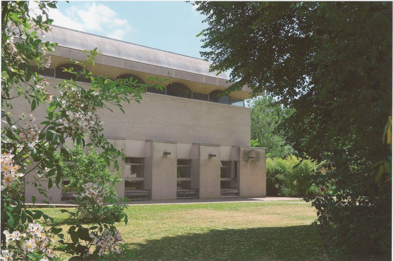
Fig. 20 | West façade of the Library as seen from the walkway. Photo: Christina Strunck
