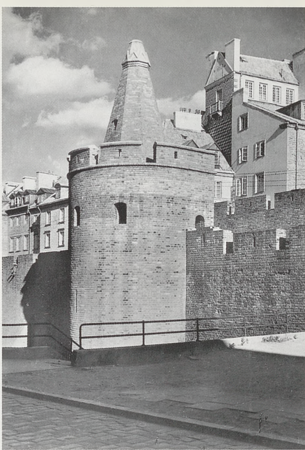
10. The tower of the outer walls in Warsaw (photo by is Pan).
