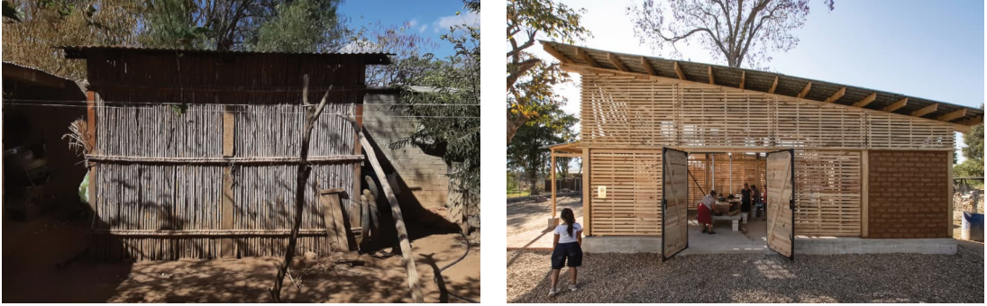
Figure 8 and 9: The kitchen as a “reinterpretation” of Quiané’s vernacular kitchens, clad in reed.
