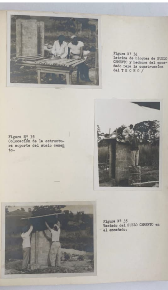
Figure 13: Application of soil cement in Chambimbal's rural housing construction, 1957.
