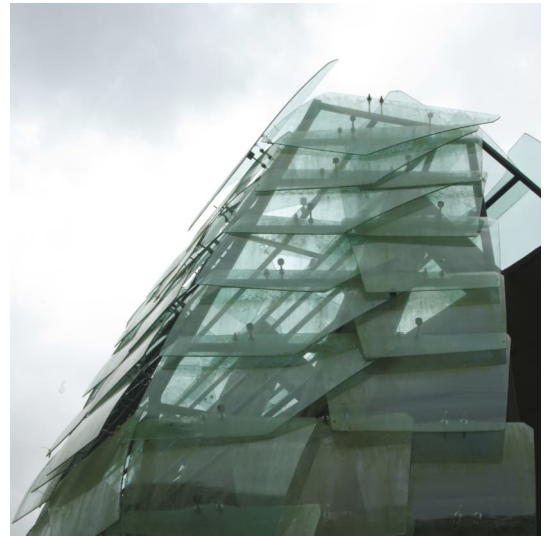
Figure 3: Scott Stafford (Rural Studio), Smoke House for Shepherd Bryant, incorporating salvaged road signs and glass bottles, built 1994 ; Forrest Fulton, Adam Gerndt, Dale Rush, Jon Shuman (Rural Studio), Detail of "Glass Chapel" made from donated car windshields, Mason's Bend, Alabama, built 2000.
