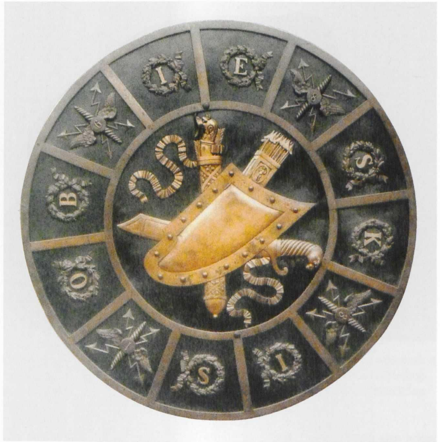
8. The second honorary shield, placed under the oculus of the Temple. In the rim of the round bronze plate was name 'Sobieski' among small trophies and royal coat of arms 'Janina': a tiny triangular gilded shield, which was fixed on hinges, that could be raised passing to the Temple hot air from the central heating stoves in narrow room within walls. This is a rare example of double function: technical and ideological of a museum object
