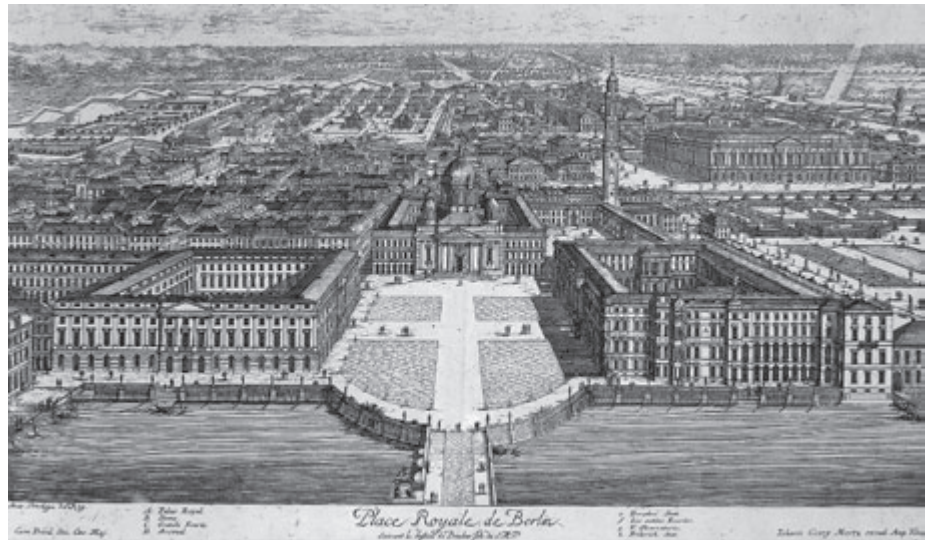
2. Jean Baptiste Broebes (c.1660–c.1720), Design for the Schlossplatz. Bird's eye view from the east with the Lange Brücke in the foreground, c.1702, engraving, 32 × 56 cm. (photo: Illustration from Jean Baptiste Broebes, Vues des Palais et Maisons de Plaisance , Augsburg 1733, Tab. 1)
