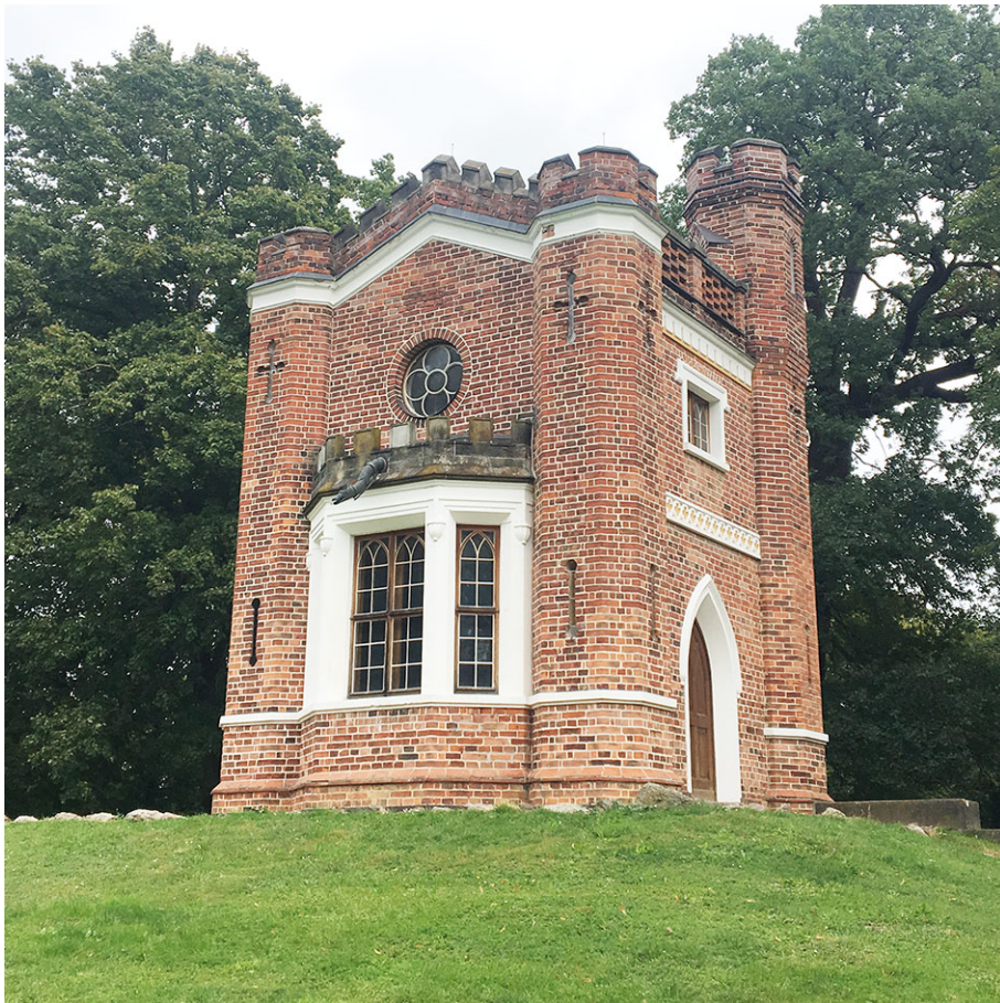
Figure 10: The West elevation of the Schlangenhaus at Luisium landscape garden.
