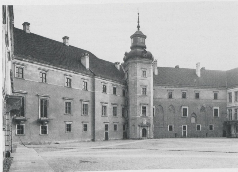
Interior of the Courtyard of the reconstructed Royal Castle in Warsaw, with the Gothic façade of the Curia Maior. Originally erected in the early fifteenth century this was covered and only revealed again in 1921.
