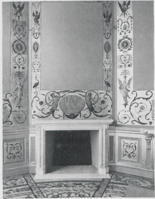
Conference Room of the Royal Castle in Warsaw at an advanced stage of the reconstruction. Clearly visible are the sections of painting rescued before the Castle was blown up.
