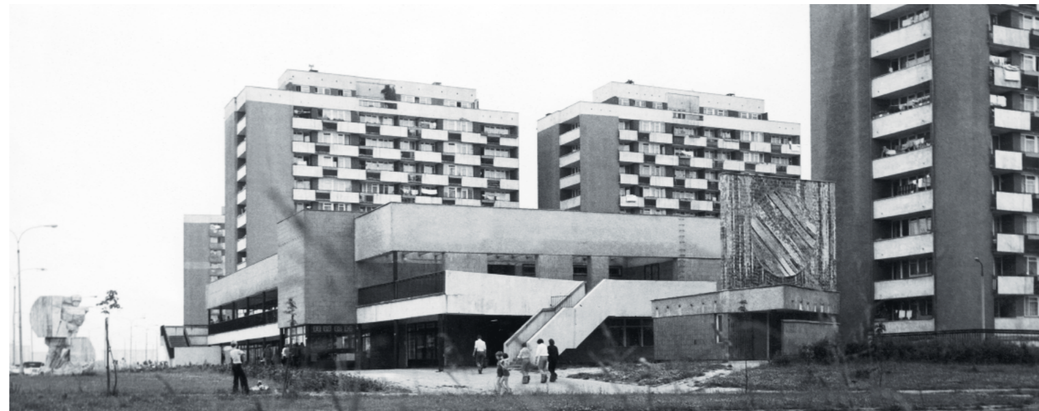
Fig. 104 View of Estate D with the mosaic-clad public convenience building, design & execution by Franciszek Wyleżuch and Stanisław Kluska, early-mid 1970s
