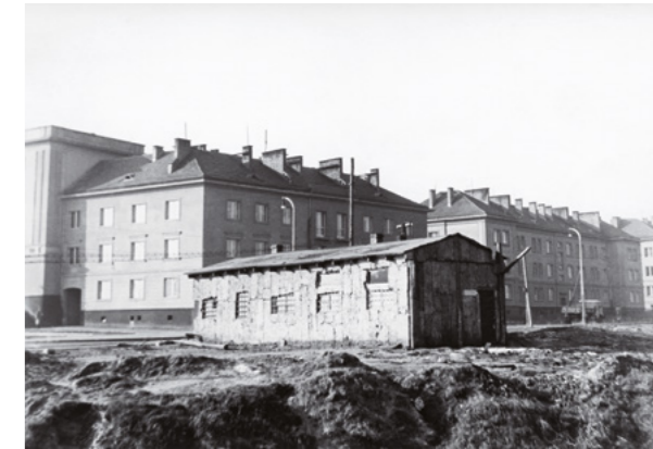
Fig. 48 Augustyn Dyrda’s studio at the former parquet workshop neighbouring Estate A near the Wilkowyja Brook, c. 1957
