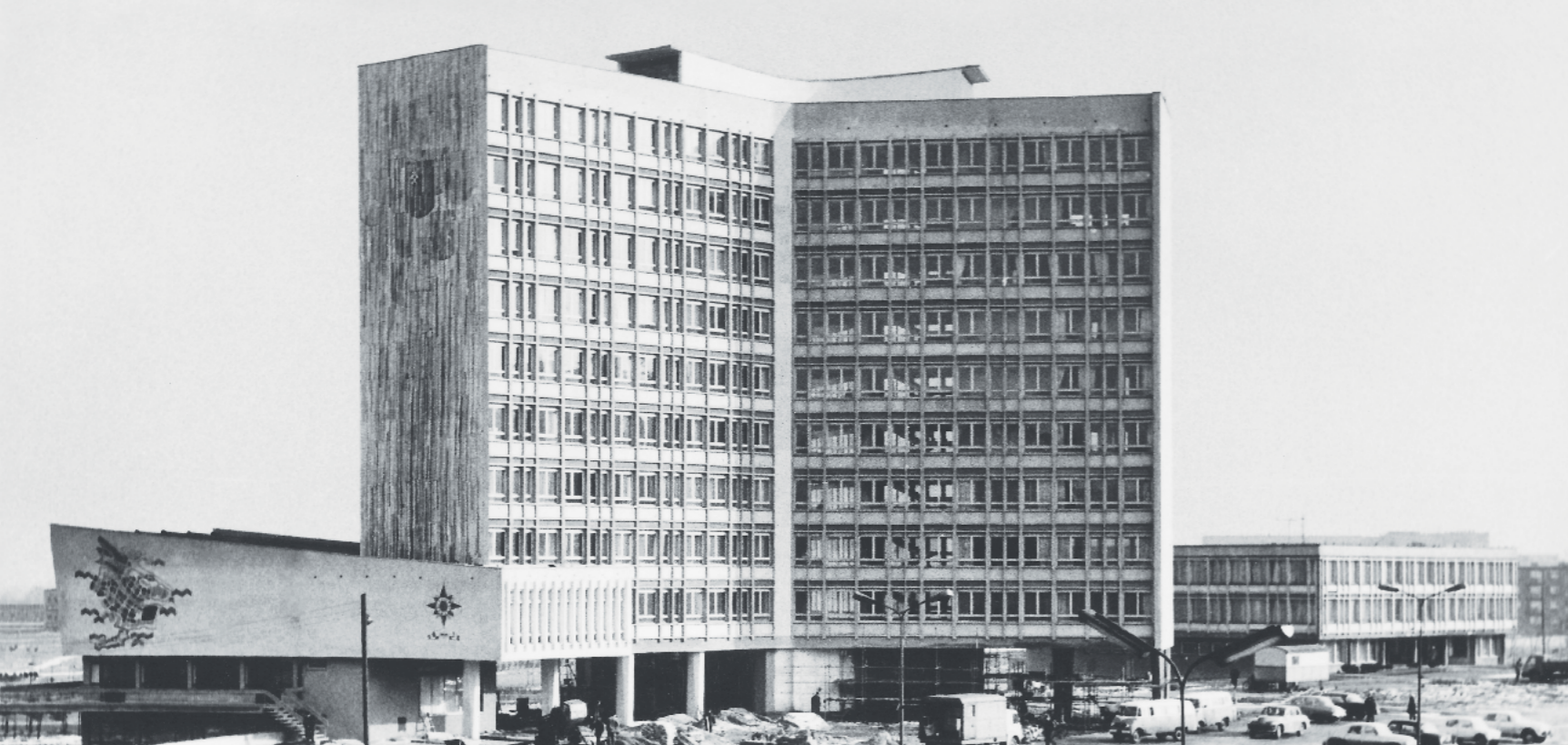
Fig. 95 Non-surviving mosaics on the City Hall's elevations, design & execution by Franciszek Wyleżuch and Stanisław Kluska, c. 1970
