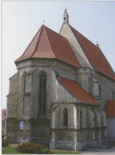
13. Stopnica: small town church of c. 1350 in Southern Poland; buttressed grey stone temple; two nave hall body, narrow choir with polygonal closure and adjacent sacristy
