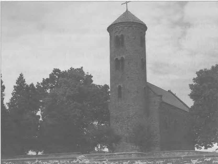
2. Kruszwica: a Romanesque basilican collegiate church; c. 1120 AD; note the “additive” manner of designing the building of simple cubes and half-cylinders
