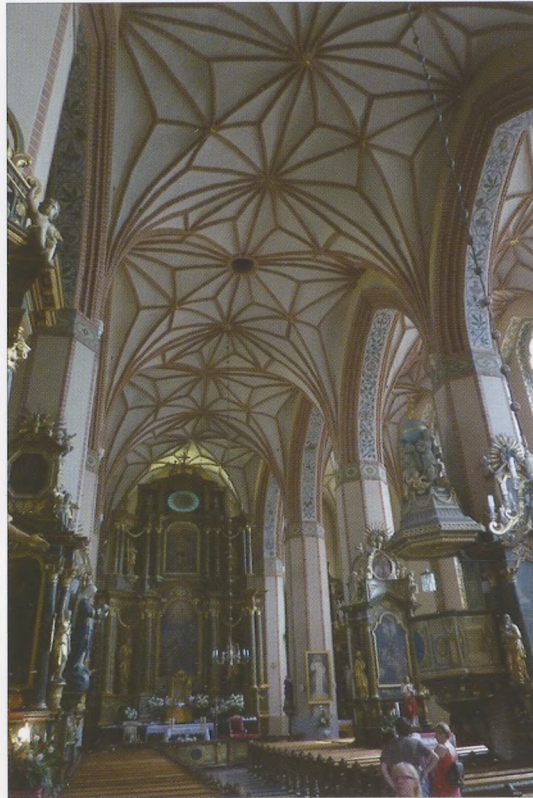
15. Reszel: interior of collegiate church in Northern Poland, c. 1475; northern Late Gothic red brick architecture; hall type church with rather heavy pillars and sophisticated “multi star” rib vaults
