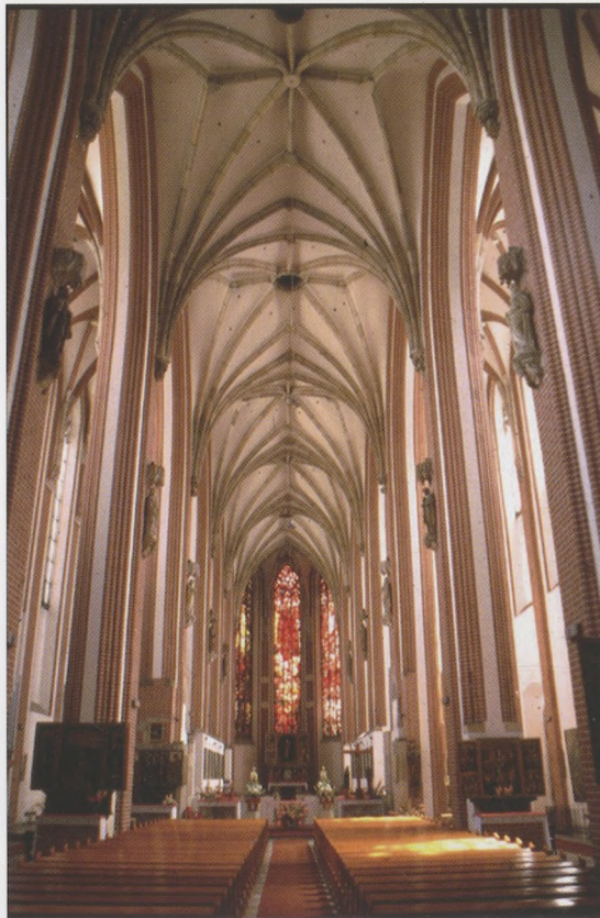
12. Wrocław: church of St Mary "on Sand Island", second half of fourteenth century; a hall system with three naves of equal height is common for High Gothic town churches
