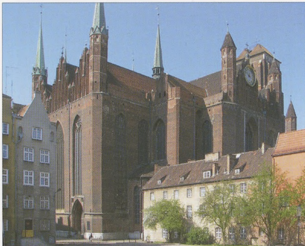
16. Gdańsk: Main Town parish church of St Mary; fifteenth century; the biggest red brick medieval temple in Europe; the construction of hall church with internal buttresses and flat outer walls, popularly named “chest Gothic”
