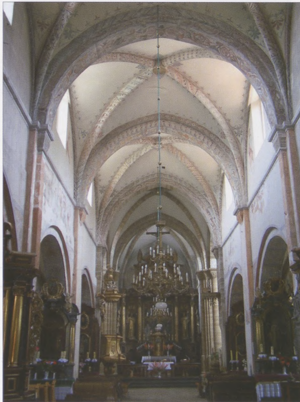
10. Koprzywnica: monastery church of Cistercian Order, c. 1220, interior; construction system with rib vaultings distinctly divided into bay canopies is typical for Early Gothic style
