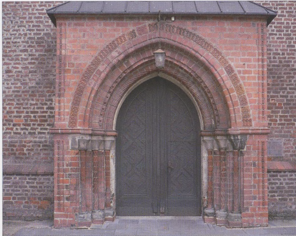
11. Poznań: main entrance to the town church of Dominican Order, c. 1240; however built of brick, with moulded ceramic decoration, the detail still shows the traces of Romanesque style
