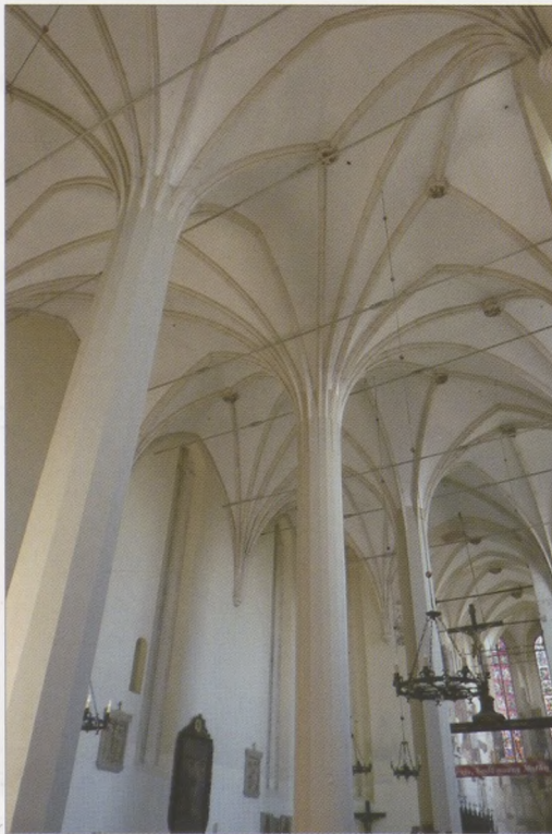
14. Wislica: interior of collegiate church of c. 1360; the complex "star" rib vaultings, resting on slim polygonal pillars take independent position to the interior walls, giving the impression of unified internal space
