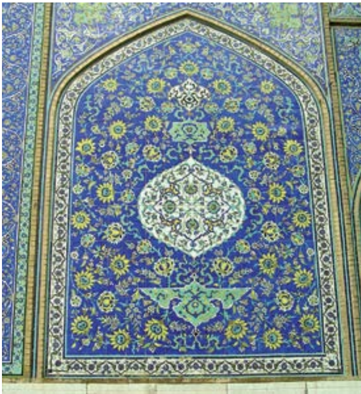
III. 3. Masjid-i Sheikh Lutfallah. Ceramic panelling on the left façade wall. Haft rangi polychrome ceramic painting, detail; phot. T. Starodub
