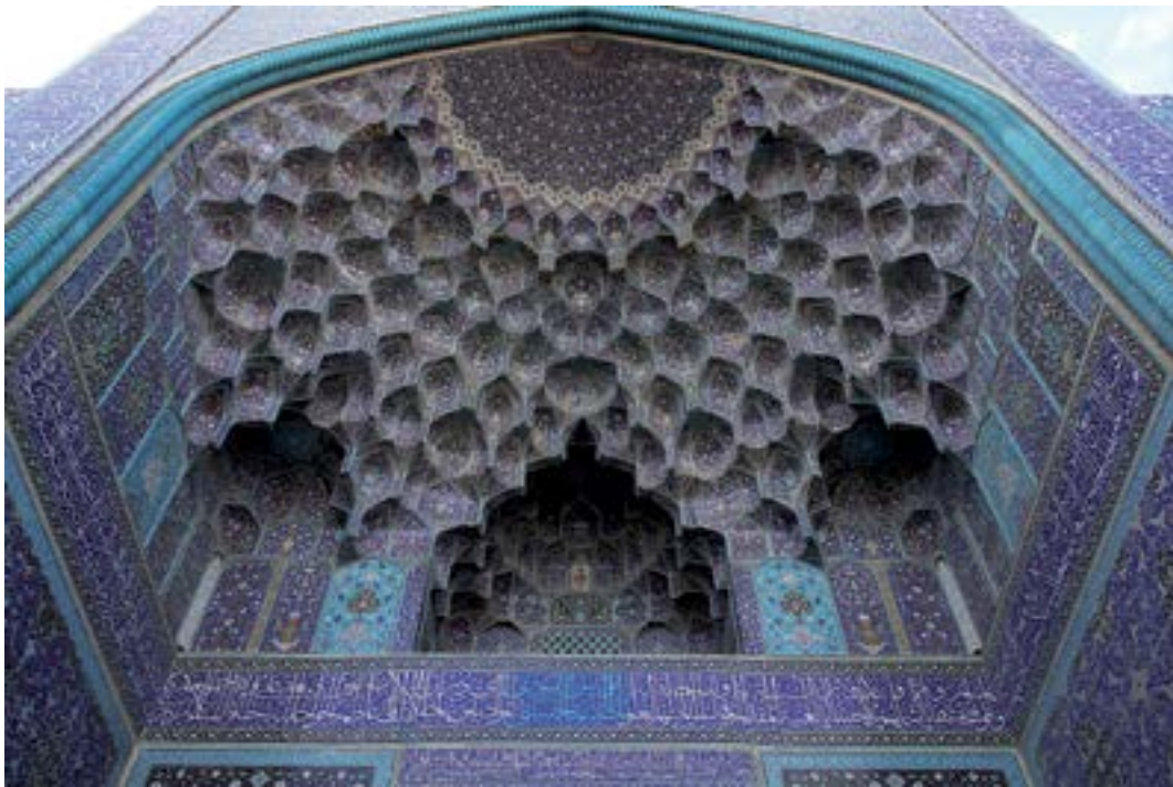
III. 4. Masjid-i Imam (Shah mosque). Muqarnas (stalactite) vault of the entry pishtak . Cut-tile mosaic; phot. V. Pappe
