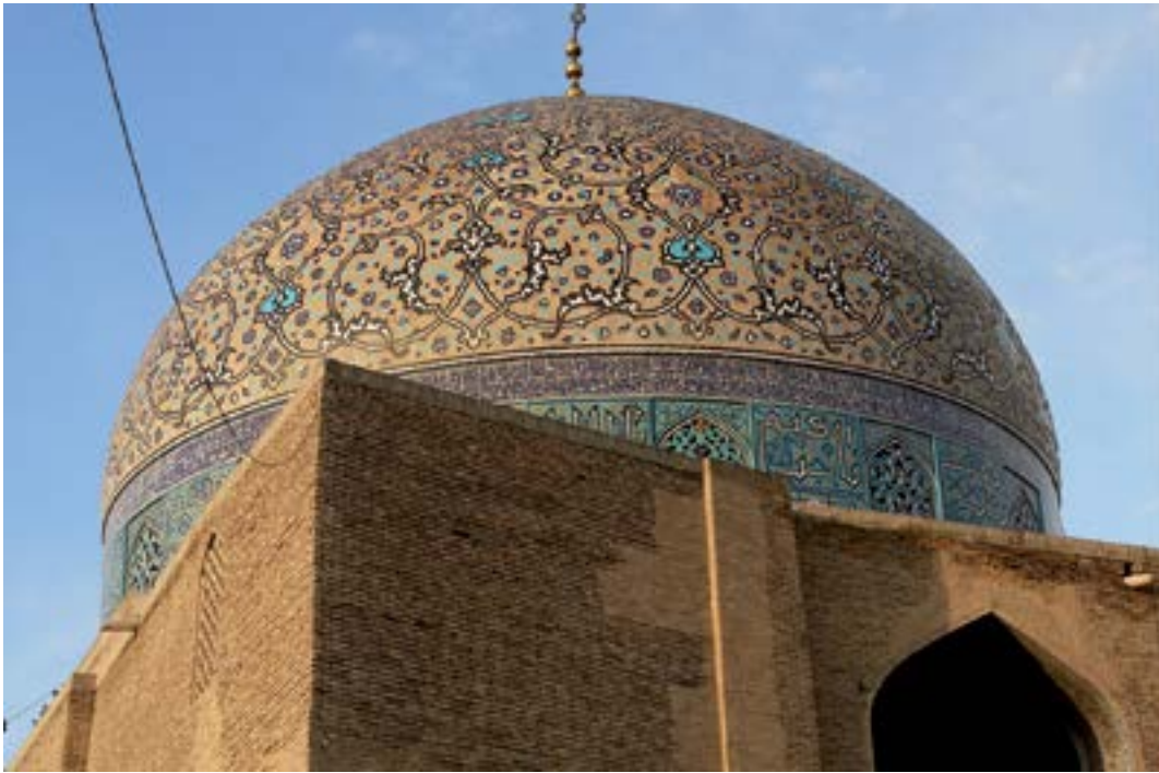
III. 1. Masjid-i Sheikh Lutfallah. The Dome outside ceramic decoration. Kashi-ye mo'arra (cut-tile mosaic or inlaid tiles); phot. Vadim Pappe
