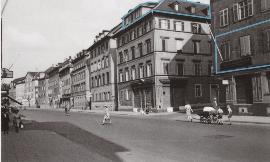
Street view with the two buildings at Hauptstätter Strasse 51B and 53A in Stuttgart, photograph, 1942, Stuttgart Municipal Archives FN250-1399StadtASgt. – From 1919 until 1930, until his mother's death, Camille Graeser lived on the fourth floor at Hauptstätter Strasse 51 ½ (later 51B), in an attic flat. Between 1928 and 1930 he also had his studio here. His aunts Marie and Sophie Cailloud lived next door at no. 53A. They earned their living as dressmakers and with a sewing school.
