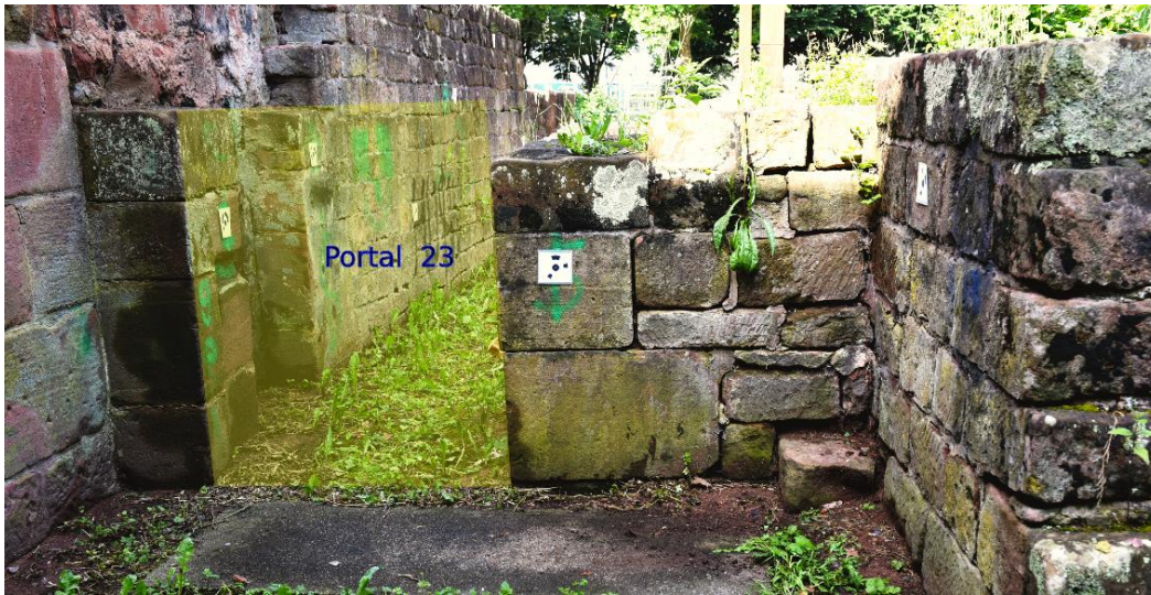
Figure 21: Portal 23 into corridor between the chapel and the curtain wall.
