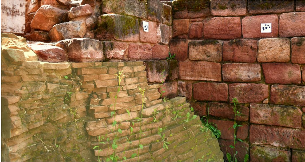
Figure 23: Natural rock outcrop (highlighted area) between the main hall and the chapel.
