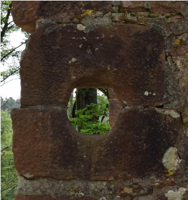
Figure 44: The restricted view of the southern gun port facing the eastern wall of the storehouse.
