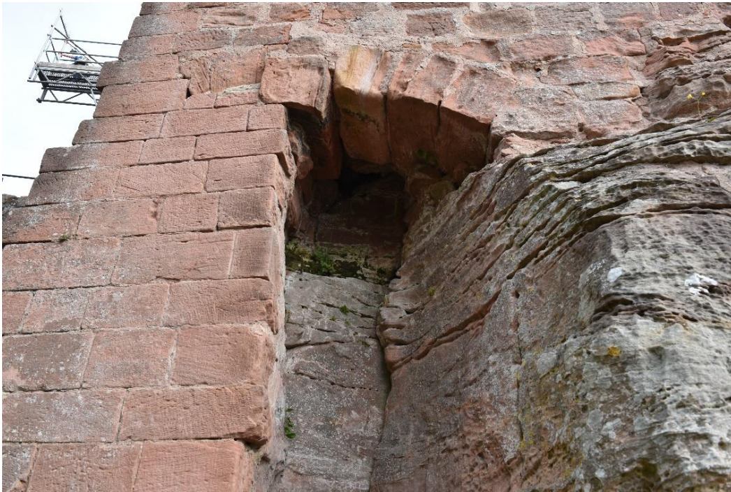
Figure 41: The support arch on the western wall of the keep.
