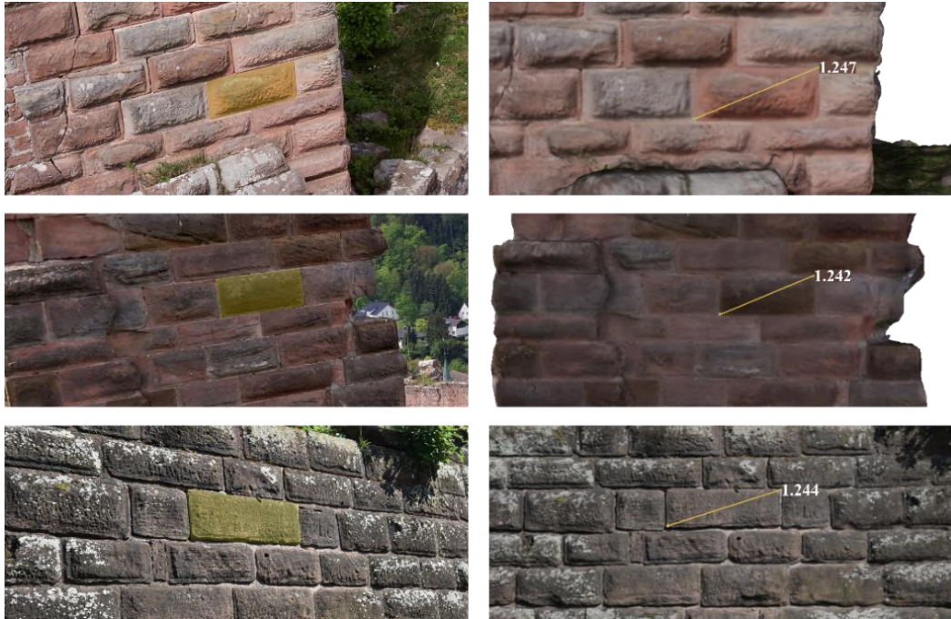
Figure 36: Comparison of embossed ashlars at Castle Hohenecken and the Palace of Lautern. Note that the discrepancies in sizes are within a margin of five millimeters.
