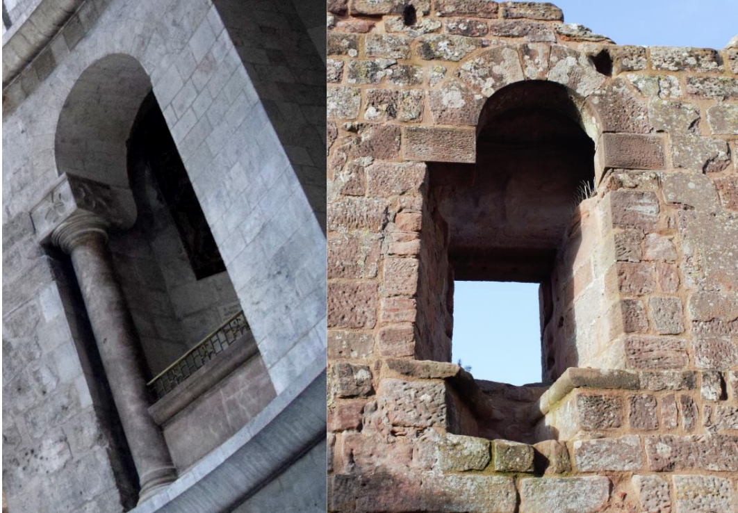
Figure 62: Comparison of arch from Window 12 and an arch from the Anastasis Rotunda in Jerusalem.
