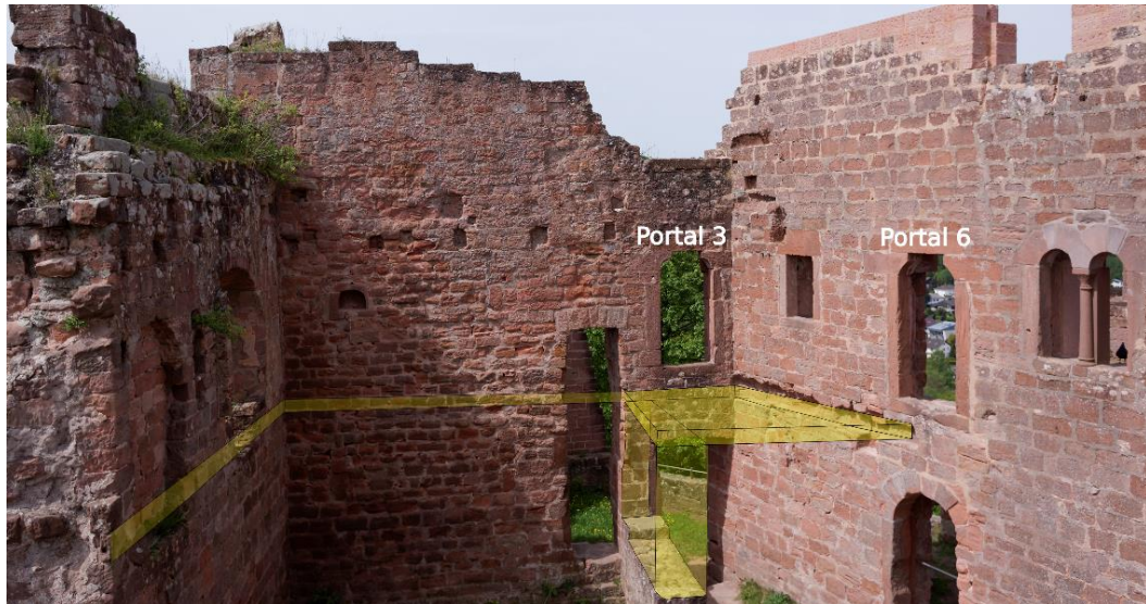
Figure 46: Hypothetical placement of mezzanine balcony connecting Portals 3 and 6. 1175
