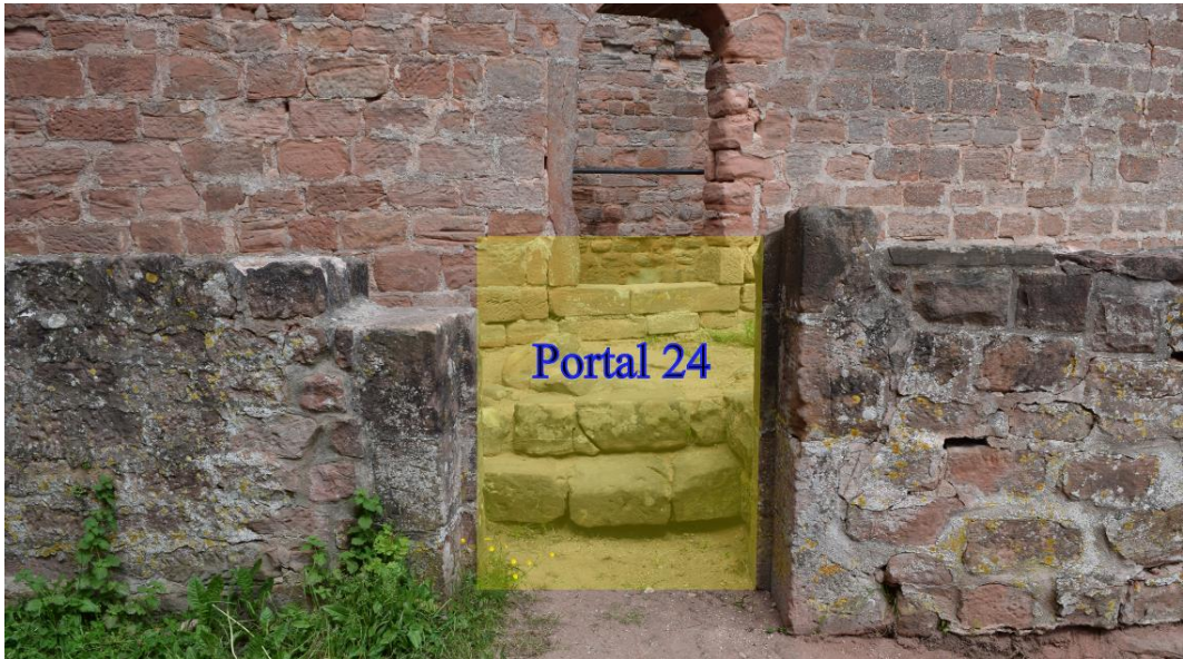
Figure 50: Portal 24 located in the northern wall of Inner Chamber A.
