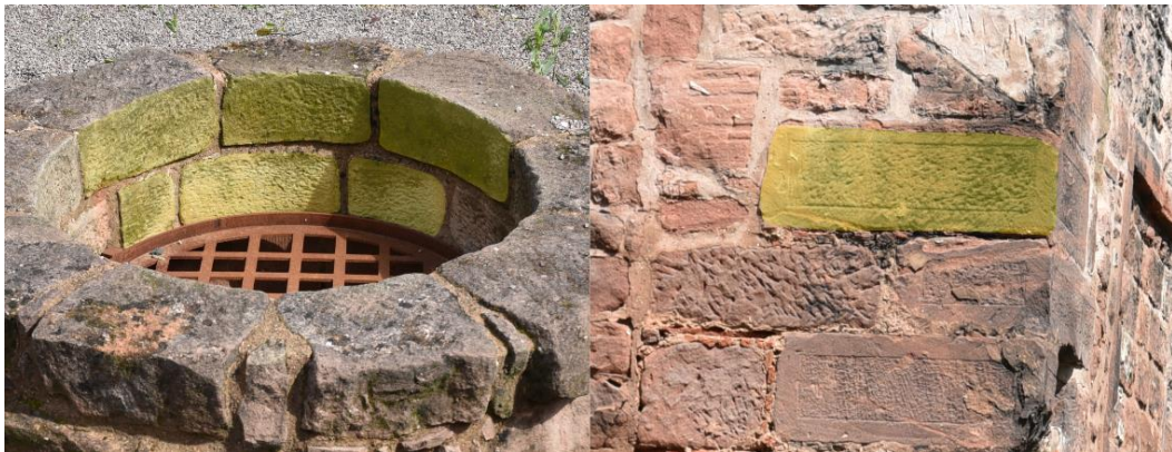
Figure 24: Comparison of the stone profiling within Well 2 (left) and the surface of Inner Chamber D (right).
