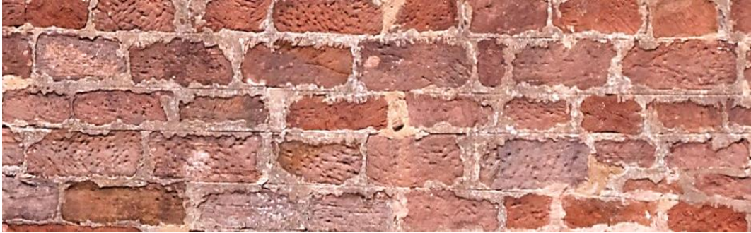
Figure 56: Traces of pietra rasa plaster on the southern wall of Inner Chamber C between levels two and three.
