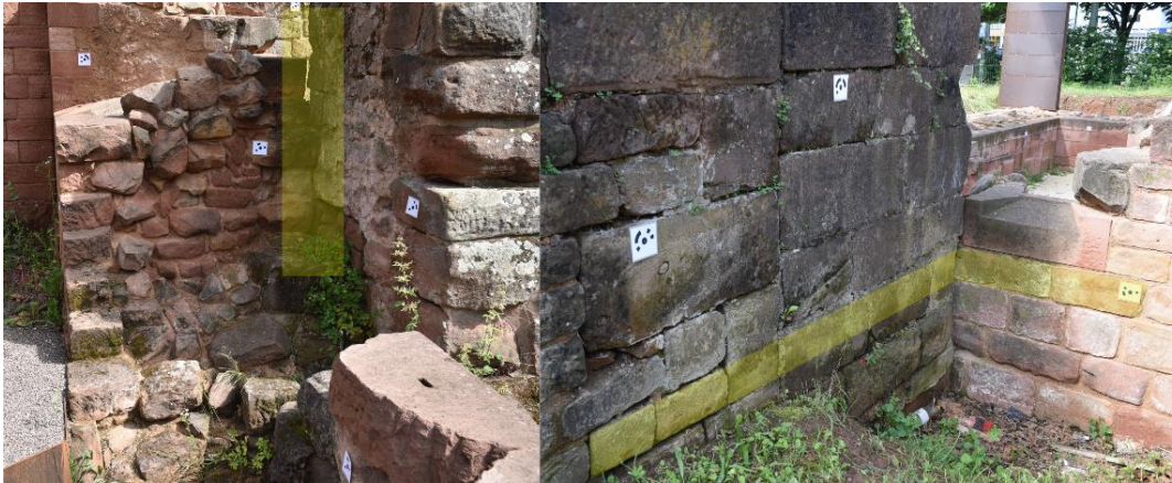
Figure 27: Connection of the Curtain Wall to the Main Hall (left) and continuation of stone courses from Salian Ward Wall to the Main Hall (right).
