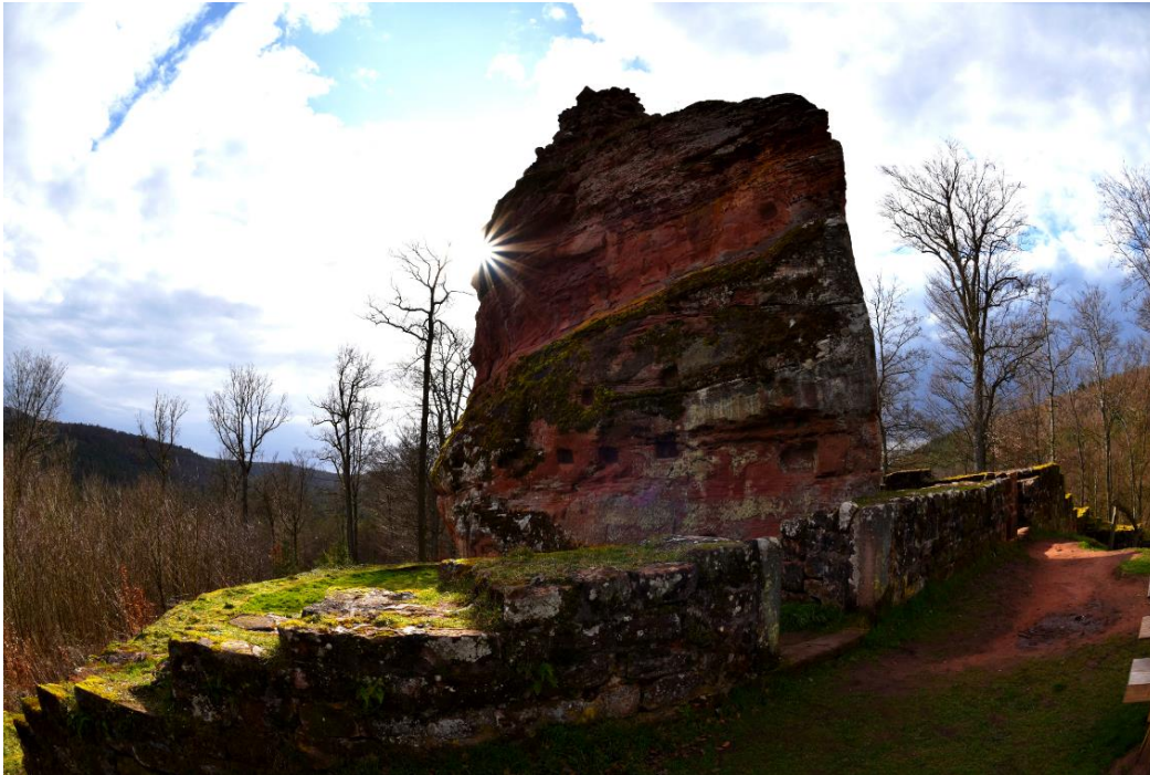
Figure 64: View of the separating wall from the south.
