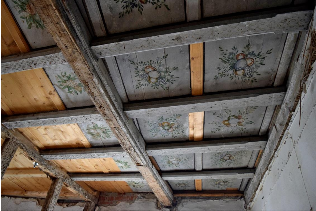
Figure 48: Ceiling lattice at Castle Colditz. Note the different levels of boards.
