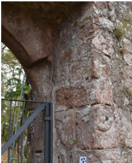
Figure 34: Inside of Front Gate. Note the segmented arch behind the rounded arch on the façade.
