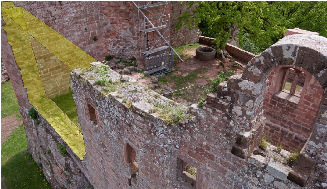
Figure 42: Hypothetical attachment between northern wall of the keep and the shield wall. 1163
