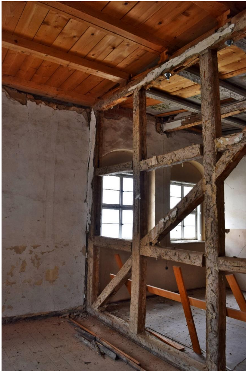
Figure 49: Half-timber construction for interior wall at Castle Colditz.
