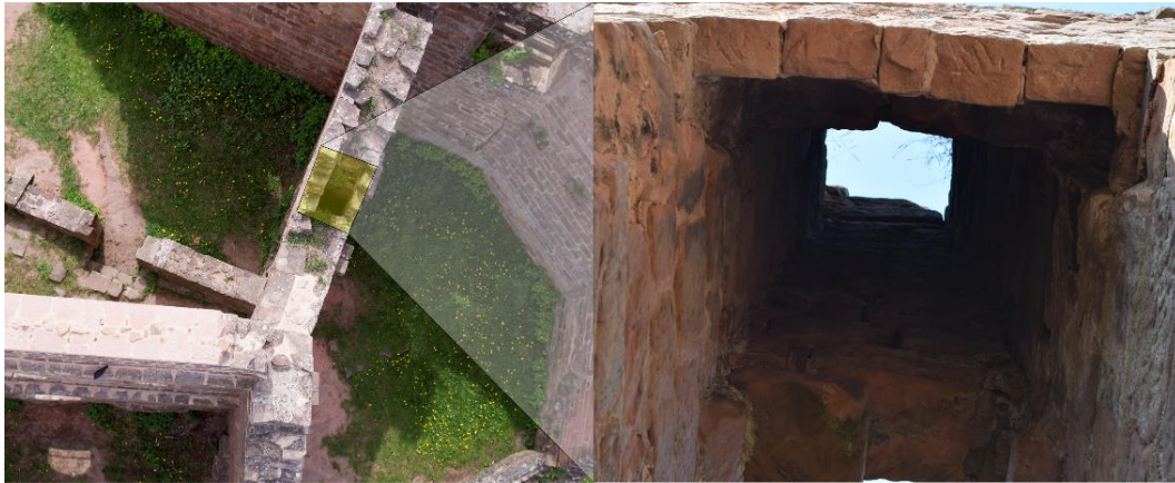
Figure 47: The opening of the service lift within the wall, from above (left) and below (right). 1178
