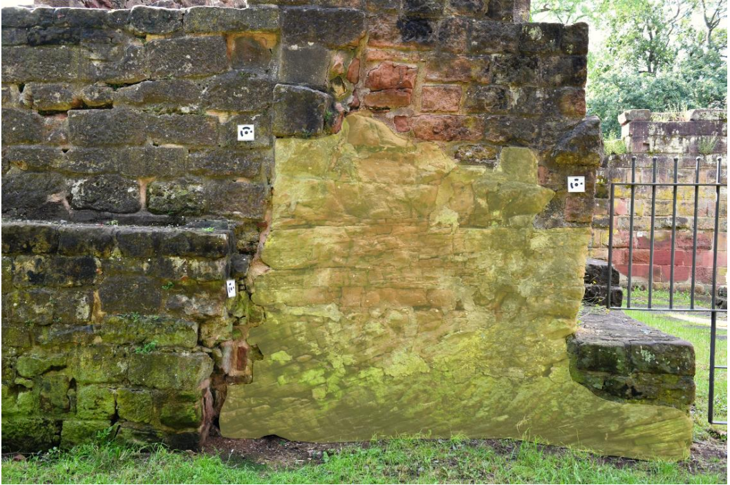
Figure 29: Natural Rock at the northwestern corner of the eastern Curtain Wall.
