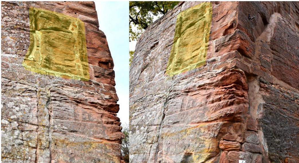
Figure 39: Connection point of the walkway between the shield wall and storehouse, in yellow.
