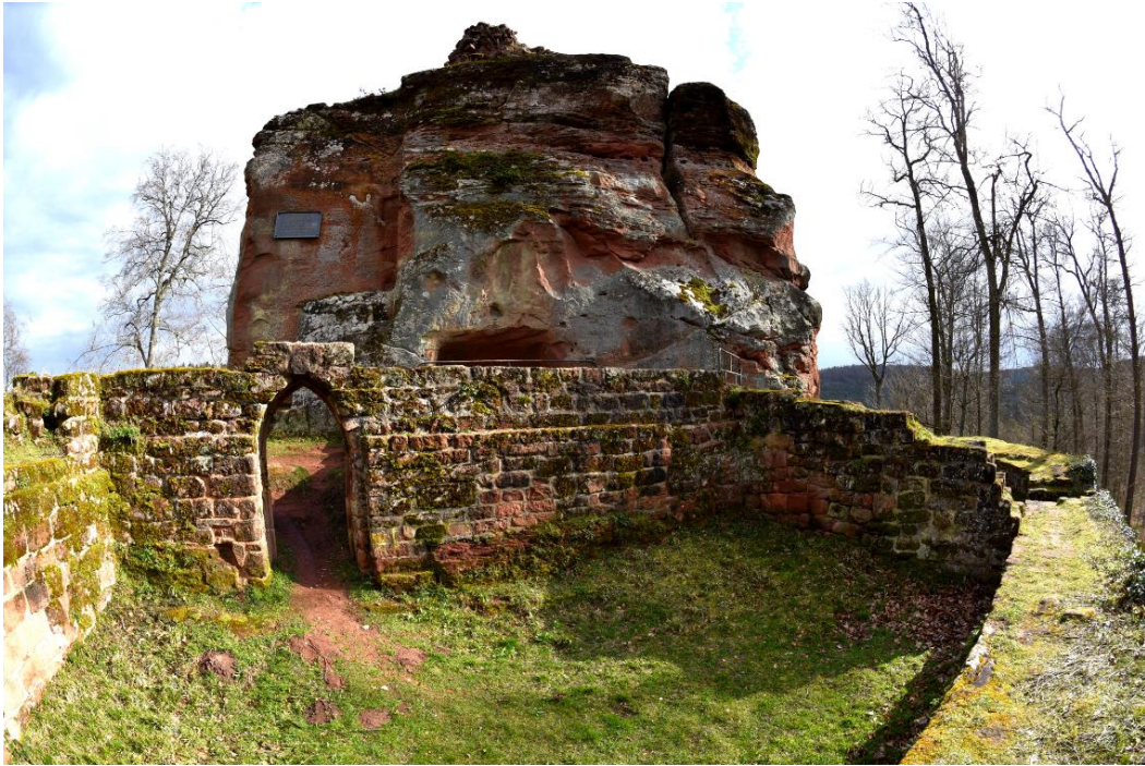
Figure 68: View of Inner Chamber F from the northwest corner atop the separating wall.
