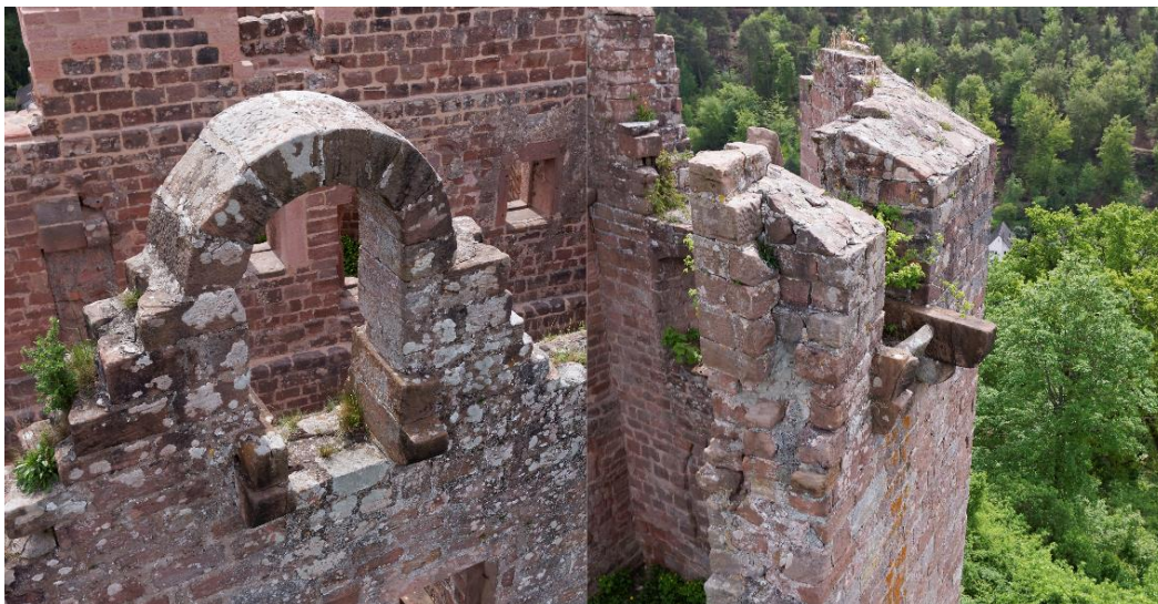
Figure 63: Comparison of the stone corbels of Garderober 4 (left) and 2 (right). 1198
