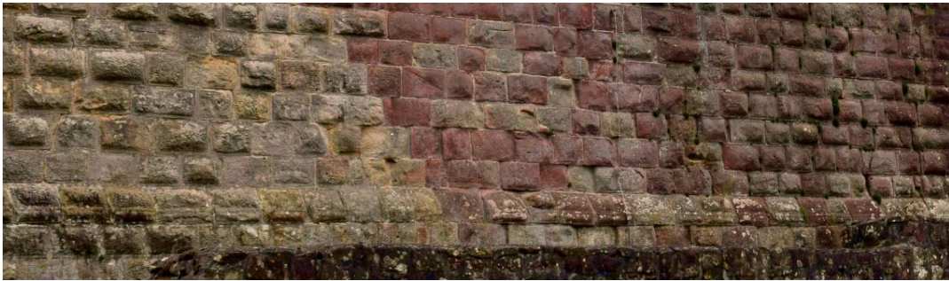
Figure 12: Embossed ashlars at the base of the tower of Castle Landeck.
