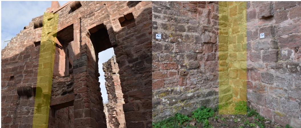
Figure 57: Connection of the stones of the eastern wall of Inner Chamber B with the southeastern corner of Inner Chamber C (left) and the southern wall of the keep (right).
