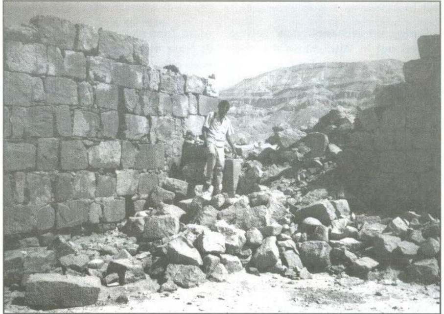
A view of part of the standing remains at Qasr Umm Ratam.
