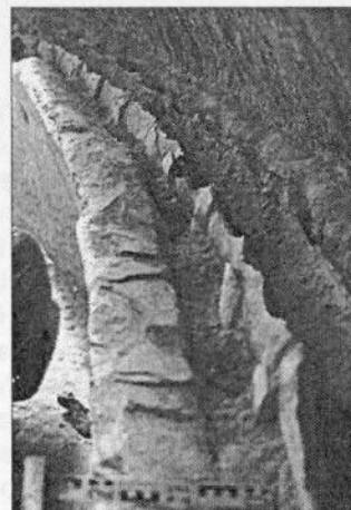
Fig. 7: Section of the terracotta pipeline along the northern cliff of the Siq in sector 21. At the joints the position of the single elements is fixed with shards from broken pipes.
