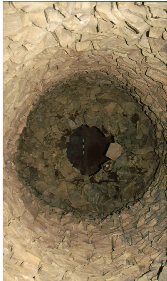
Fig. 38. View in tomb Shi2 from above through the upper vault into the collapsed lower vault.
