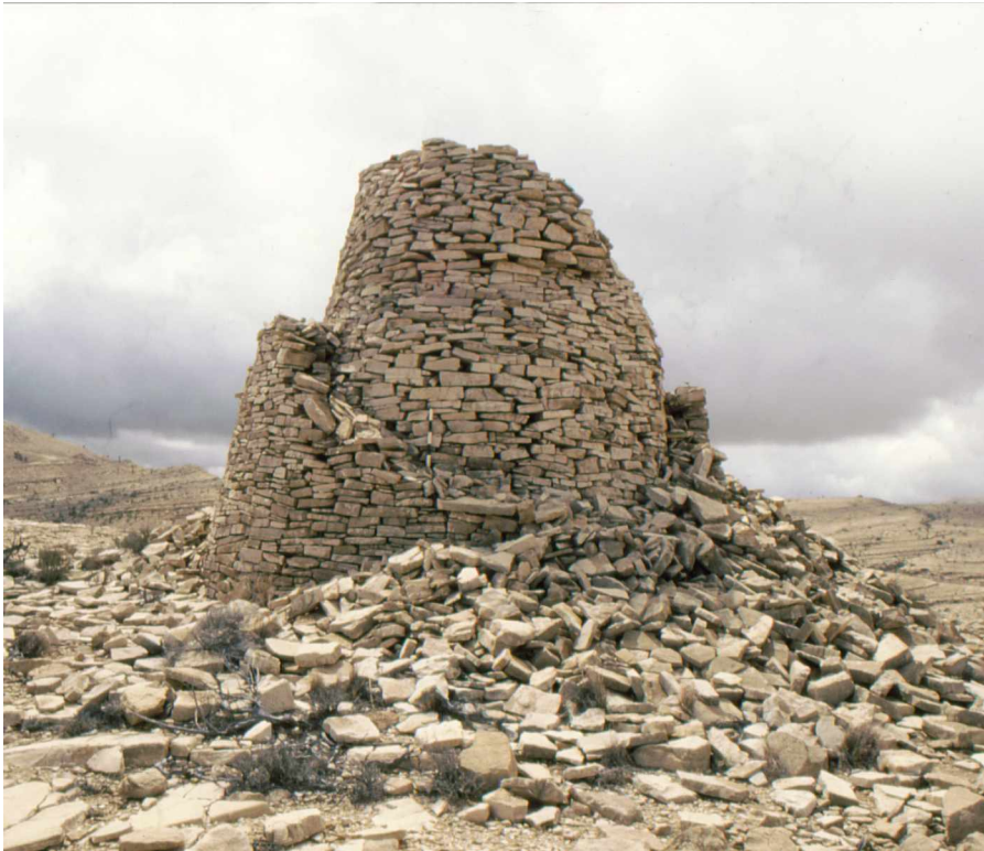
Fig. 49. Tomb Shi21 showing the double wall construction.
