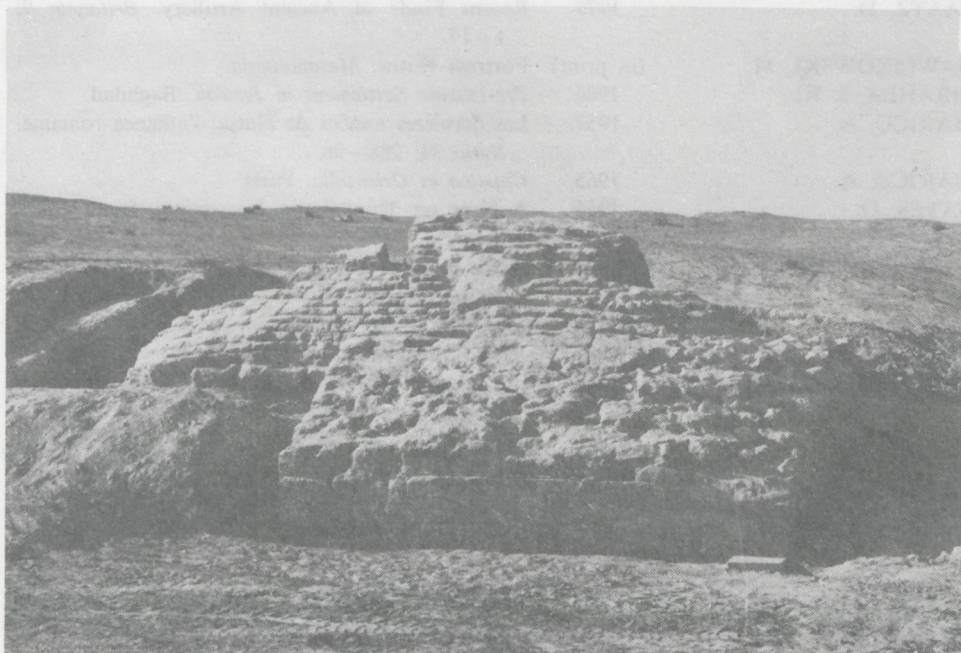
Fig. 7 The corner tower of the discovered old rampart. (Photo by M. Gawlikowski)
