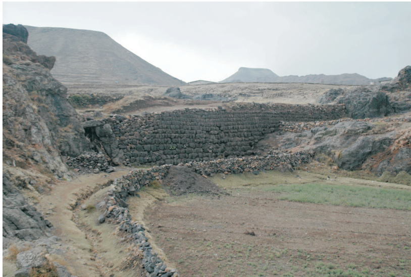
Fig. 11 Zafar/al-Shugag sadd z326 toward the north-east. An ancient well is located on the left (north) side of the dam.
