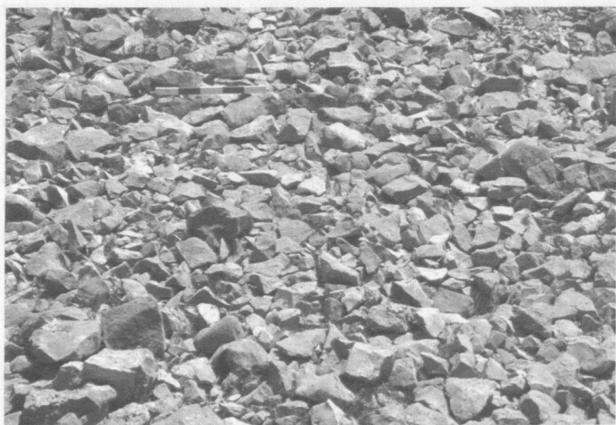
Fig. 11 – Close-up view of the surface of the flake embankment in fig. 9, showing the particularly limited range of sizes and shapes of the limestone flakes. Bar scale in top left part of the picture is 50 cm.
