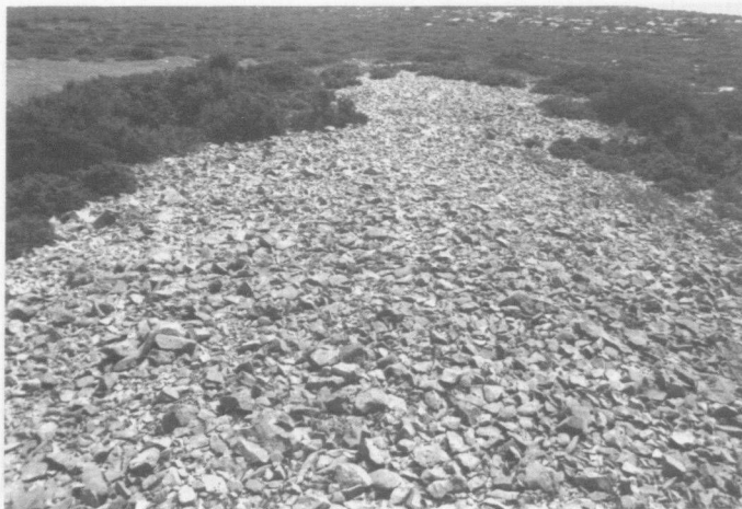
Fig. 9 – Quasi-linear embankment, southwest of Didyma, consisting of relatively equally sized, sharp-edged flakes of limestone. The embankment is some 6-8 m wide and up to 3.5 m high, shrubs of macchia obscure the sloping sides of the embankment.
