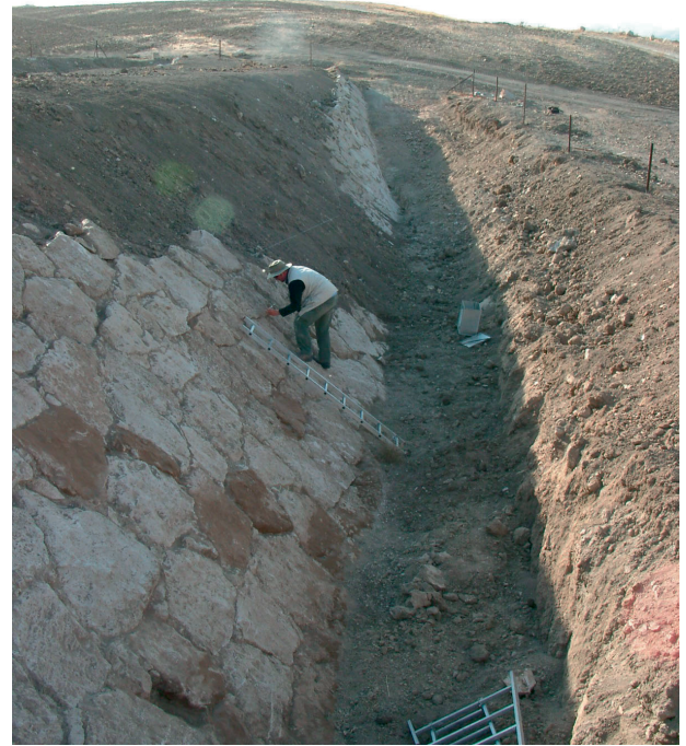
Fig. 6. Excavation of the dam.
