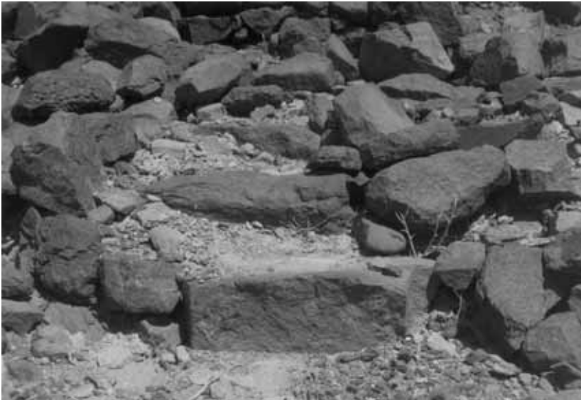
Fig. 46. Steps, probably part of a connecting path on the southern side of the fortification.
