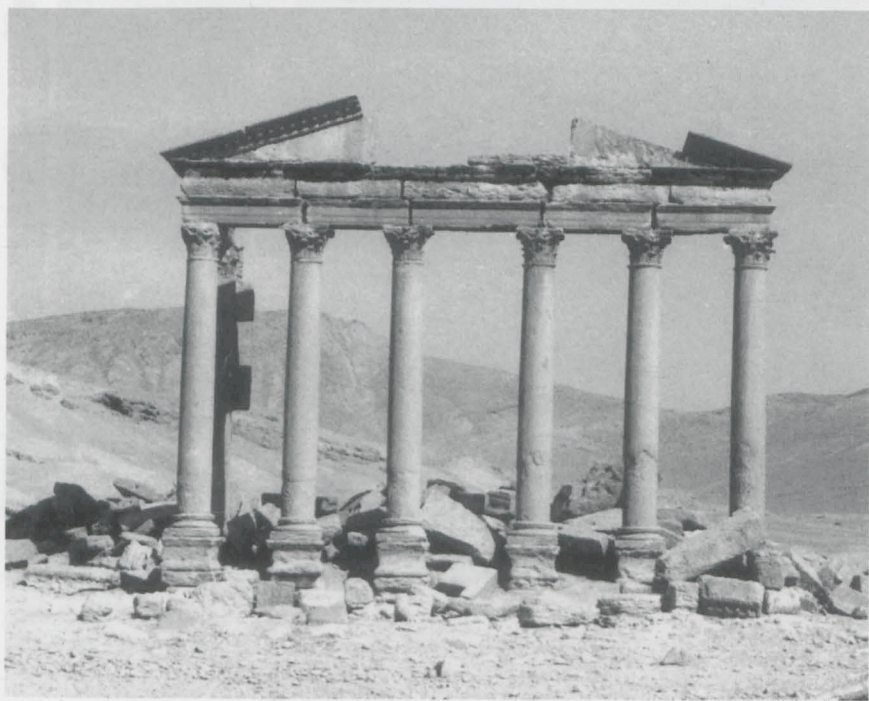
Fig. 12. The porch of the funerary temple no. 86 (before restoration)
