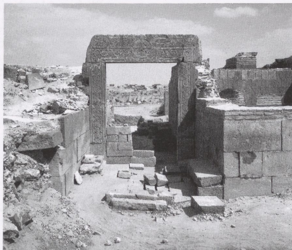
Fig. 3 Androna, Kastron: the western entrance gate.
