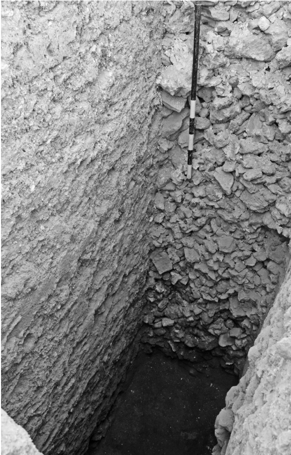
Fig. 8. Room Q: The southern subterranean foundation wall (left) of the room with a 'couloir-type' stone alignment (back) and a retaining wall (right).
