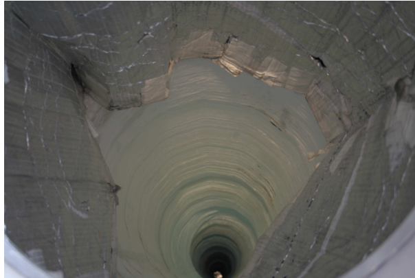
Figure 5.2.: A 2.5 km deep hole drilled to accommodate a new IceCube string. Pressurized hot water is used to melt the ice. Photo: R. Maruyama
