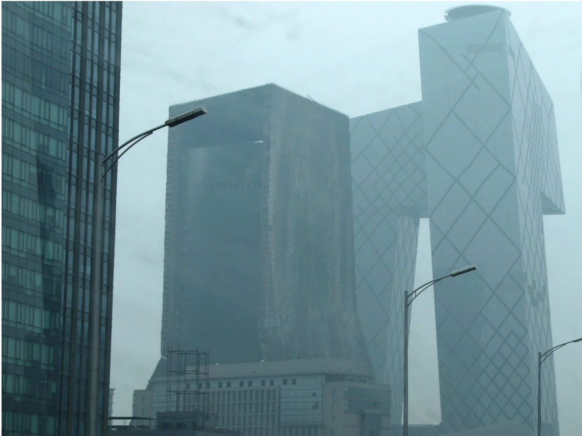
Figure 36: China Central Television Tower after the fire, April 2009
