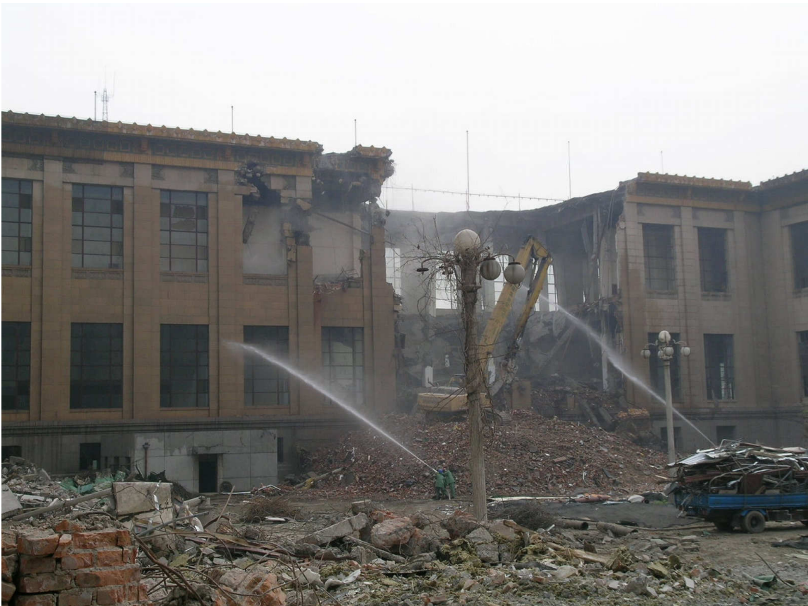
Figure 10: National Museum of China, deconstruction of the eastern building section, April 2007
