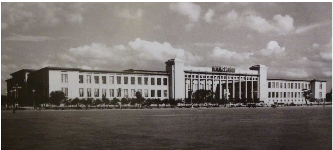
Figure 4: National Museum of China, the original main façade (1959), from Beijing shida jianzhu sheji 2002 , p. 166.
