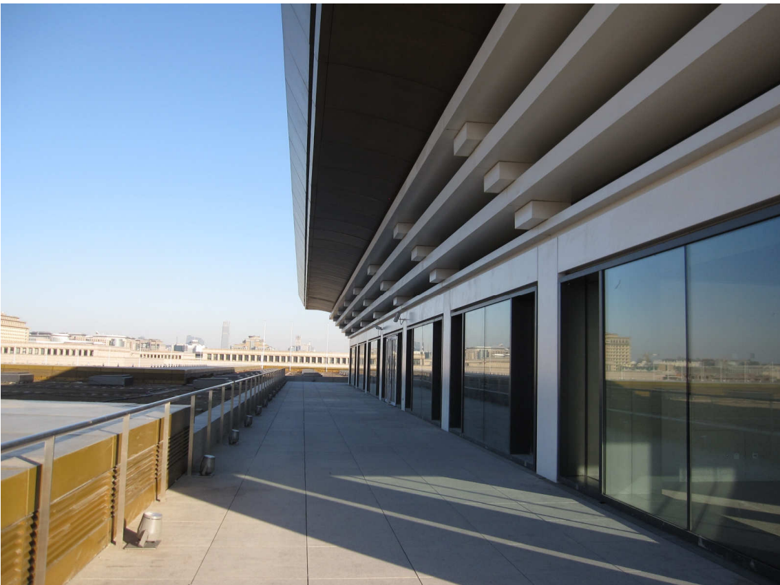
Figure 73: National Museum of China, roof terrace, January 2011
