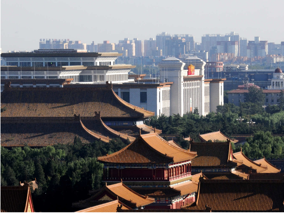
Figure 42: National Museum of China, roofscape, courtesy of Dong Qing, September 2010
