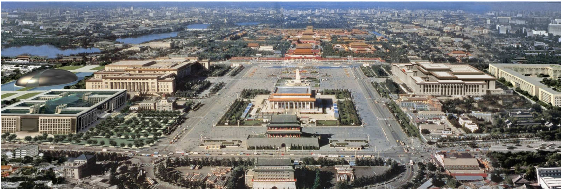
Figure 23: Tiananmen Square, National Museum of China with new design, rendering, courtesy of gmp 2004
