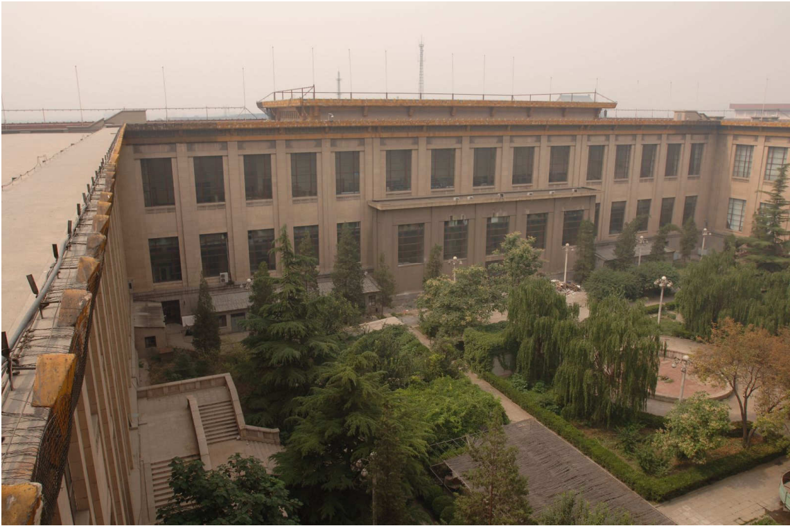
Figure 52: National Museum of China, south courtyard with planting beds, courtesy of Dong Qing, June 2006
