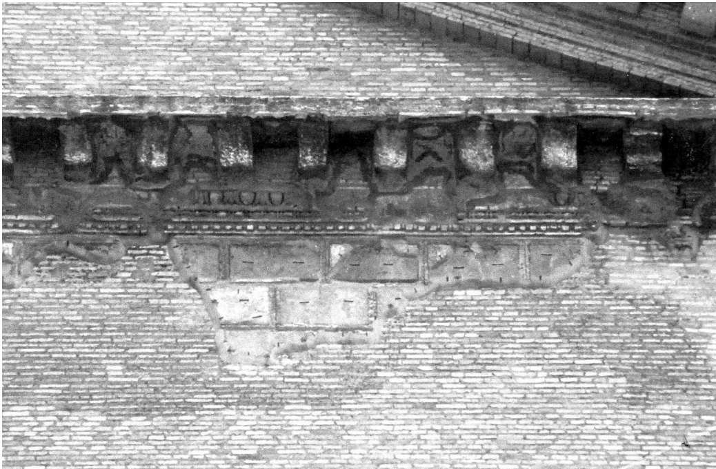
Abb. 55: Curia, Außenwandputz in Quadersteinimitation.
