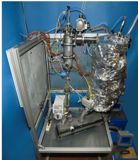
Figure 6.23: Picture of the adsorption chiller test stand.
