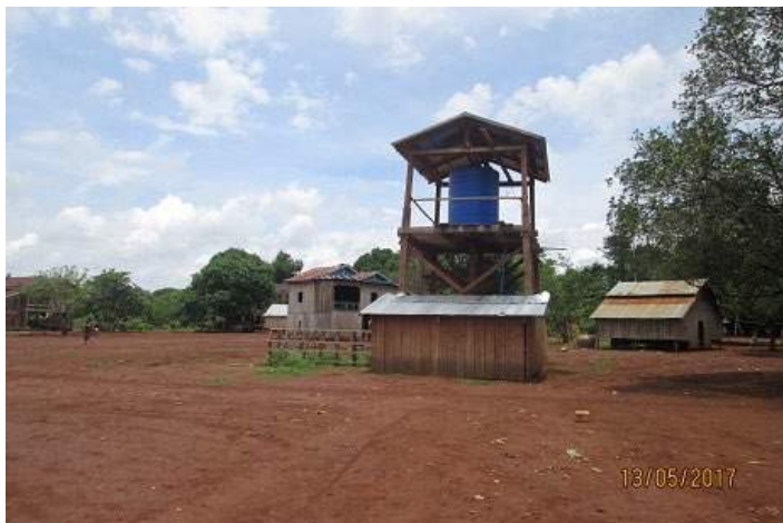
Photo 28: Water storage tank
