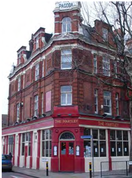
FIGURE 7.112. The Pagoda pub at 64 Tower Bridge Road, January 2007.
