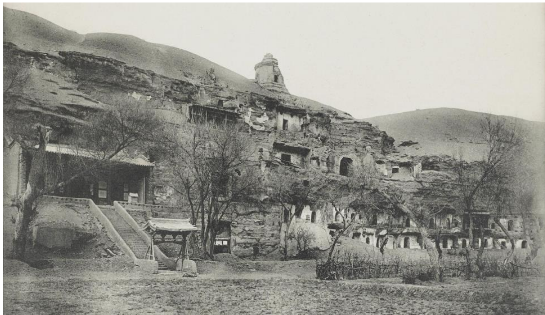
Fig. 5.1-7a. The remains of building in front of the Mogao Caves After Mission Pelliot, Les grottes de Touen-Houang (Paris. Librairie Paul Geuthner, 1920), Plate. V.
