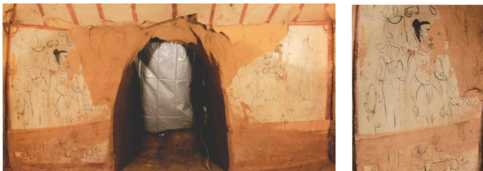
Fig. 4.1-19b A monk kneeling on a bed of ropes on the south wall of Badaliang Cemetery M1.
