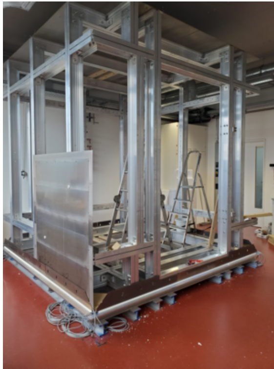
Figure 8.1.1: Internal structure of the MSR with Mu-metal plates to be attached.
