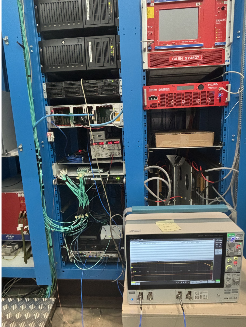
Figure 5.30: FELIX-based data acquisition rack during integration tests. The LTI (bottom) distributed the clock to FELIX, while an oscilloscope monitored the startup phase of the recovered clock at the Module Flex against the LTI reference clock.
