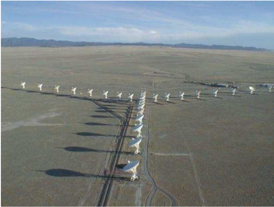
Figure 2.1: The National Radio Astronomy Observatory’s Very Large Array (VLA). The radio interferometer consists of 25 antennas, each 27 m in diameter. The maximum antenna separation (A array configuration) is 36 km. Its sensitivity corresponds to what could be achieved with a single dish 130 m in diameter. (Image courtesy of NRAO/AUI)
