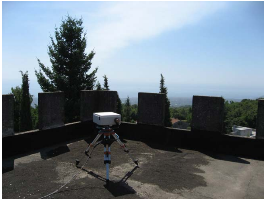
Fig. 5.26 – NOVAC mark II DOAS instrument at the site milo_tommaso_house_uhei. The instrument power is supplied by land line and buffered by an 80 Ah car battery. Data is transmitted via WLAN antenna (not shown) to a repeater site on the southern edge of the horseshoe shaped Valle del Bove (see Fig. 5.25). The volcanic plume is clearly visible in the sky over the instrument.
