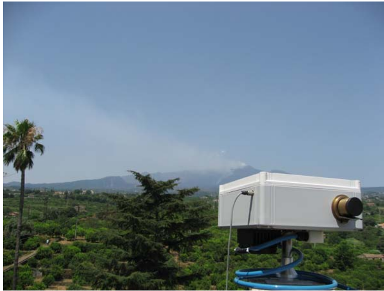
Fig. 5.27 – NOVAC mark II instrument installed at the Polizia Municipale in Giarre. Here, the instrument is mounted on a concrete wall at the base of which a second box contains an 80 Ah car battery, a charger and a timer. Again, the battery is charged by land line. The cable shown hanging out the side of the instrument is used to communicate with the temperature controller and is disconnected after successful configuration.
