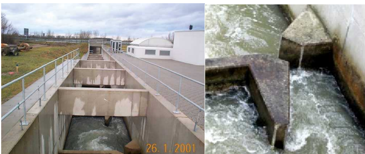
Fig.9 Fishpass in Iffezheim dam. On the right the fishpass spot (Image by Mr. Degel)
