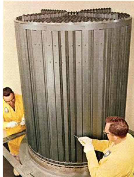
Figure 1.6: Graphite core of the MSRE at Oak Ridge.
